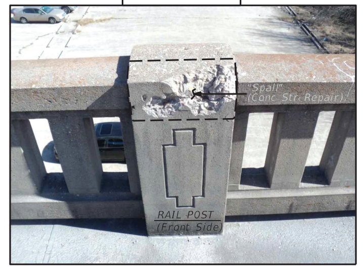
SPALL REPAIR AT RAIL POST
