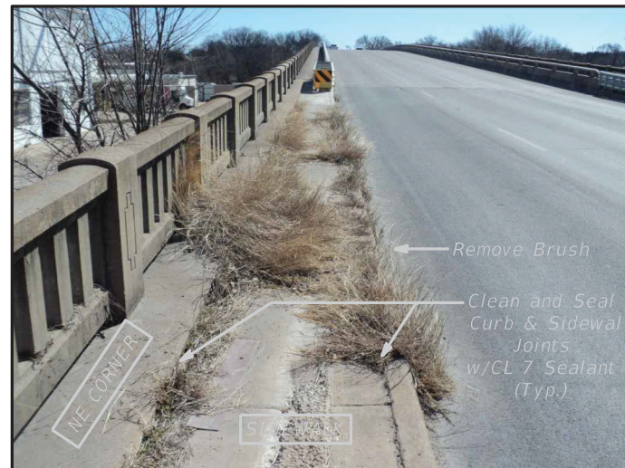
BRUSH REMOVAL AT SIDEWALKS
