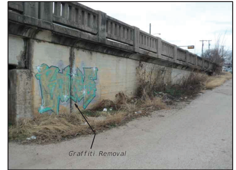
BRUSH/DEBRIS REMOVAL (SHOWING RETAINING WALL AT NE CORNER)
