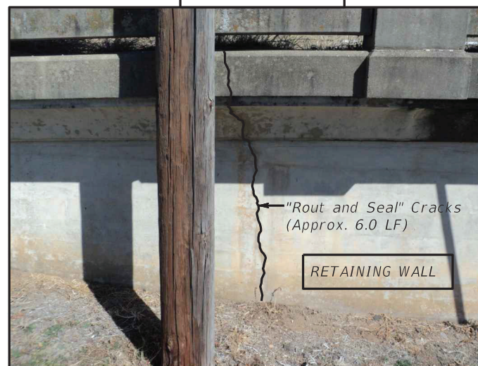
CRACK REPAIR AT NW RETAINING WALL
