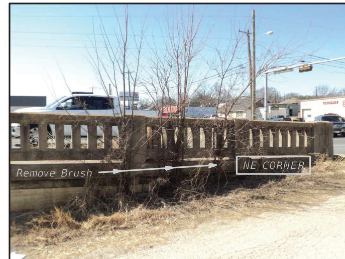
BRUSH REMOVAL AT END OF RETAINING WALL
