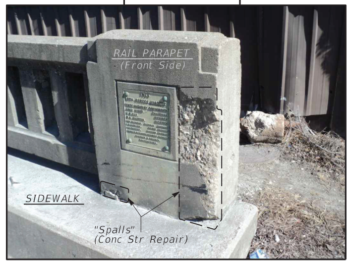
SPALL REPAIR AT RAIL END POST (FRONT SIDE)
