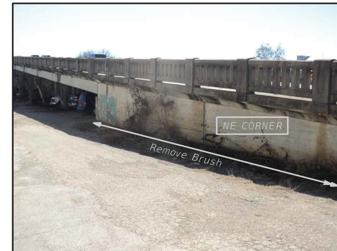
BRUSH REMOVAL AT RETAINING WALL
