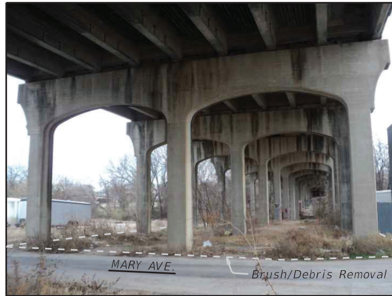
BRUSH/DEBRIS REMOVAL (SHOWING INTERIOR BENT LOCATIONS AT NORTH END)
