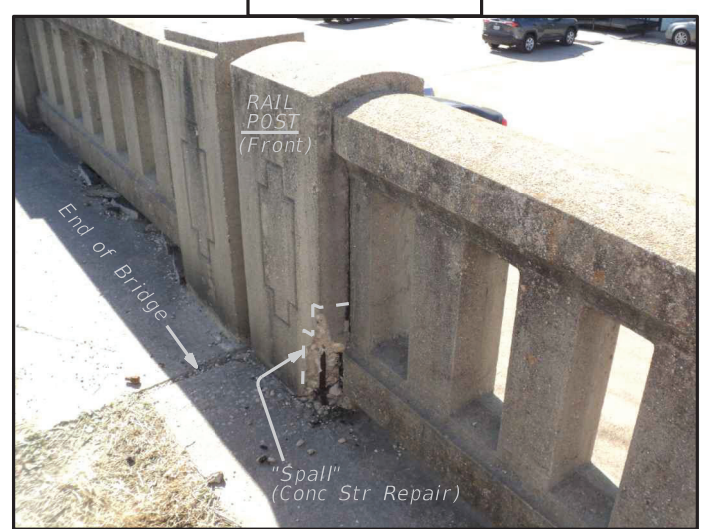
SPALL REPAIR AT RAIL POST (END OF BRIDGE)
