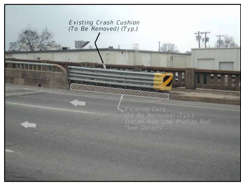
ELEVATION AT END OF BRIDGE SHOWING LOCATION OF PROPOSED LOW-PROFILE RAIL NOTE: WEST SIDE SHOWN ~ EAST SIDE SIMILAR
