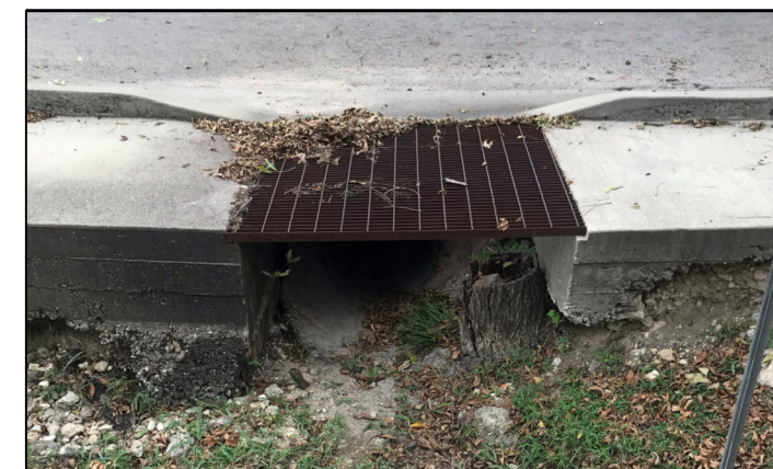
PHOTO OF REPAIR LOCATION
