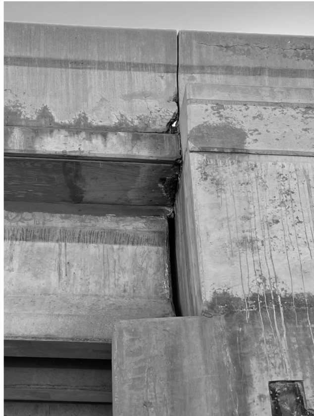
BRIDGE RAIL AT WEST END OF SOUTH ABUTMENT
