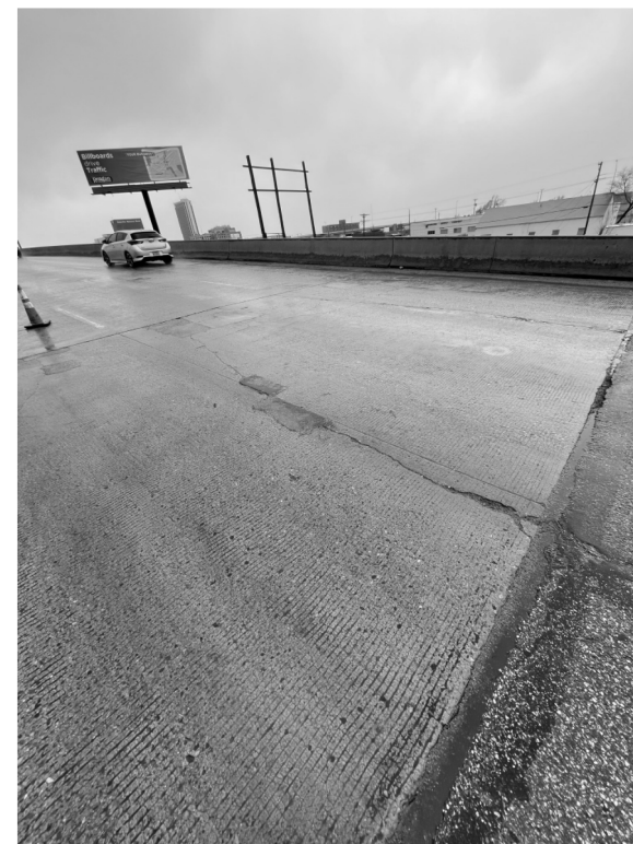
NORTH APPROACH SLAB
