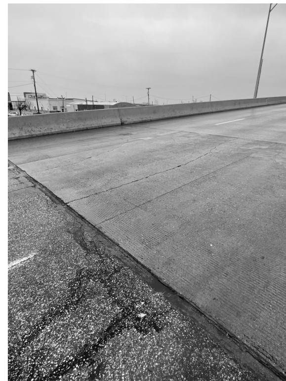
SOUTH APPROACH SLAB
