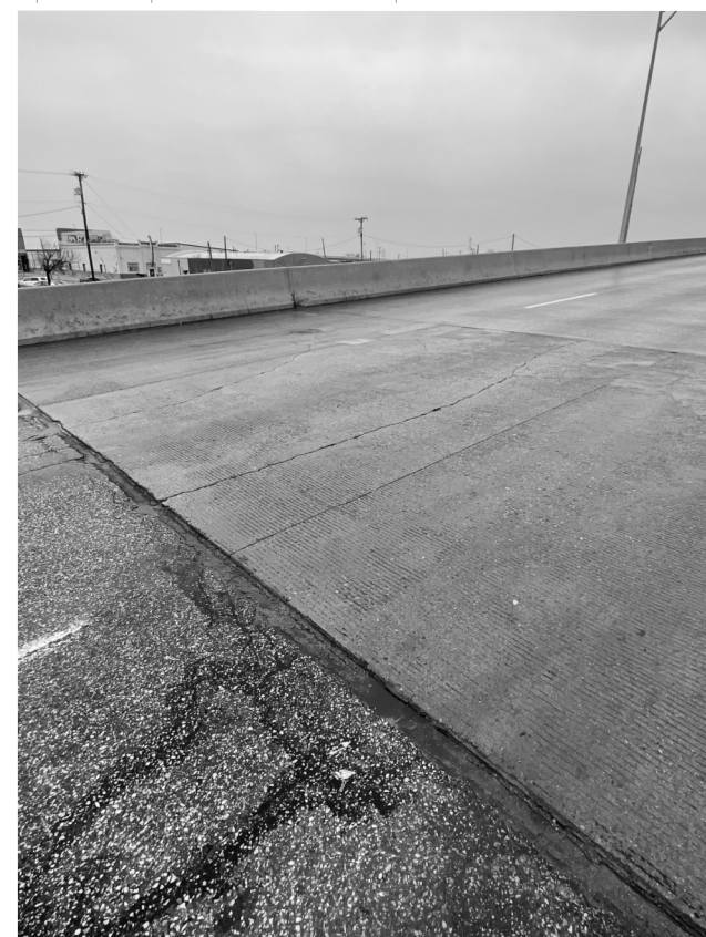
SOUTH APPROACH SLAB
