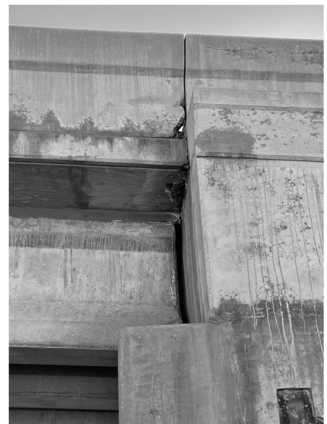
BRIDGE RAIL AT WEST END OF SOUTH ABUTMENT
