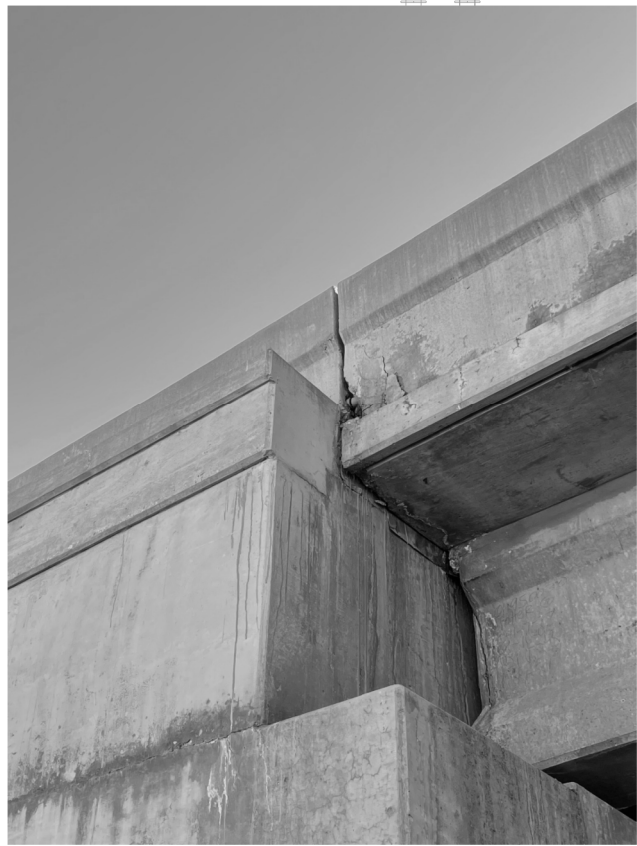
BRIDGE RAIL AT WEST END OF NORTH ABUTMENT
