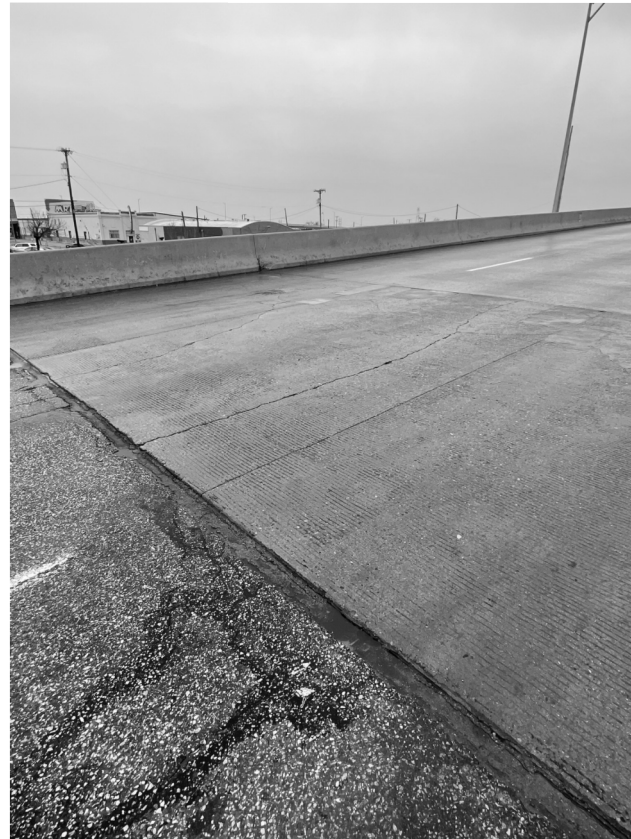
SOUTH APPROACH SLAB
