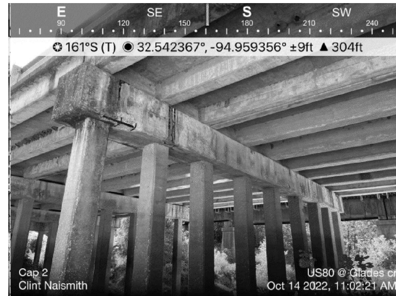
TYPICAL SPALL (SBI) PHOTOS
