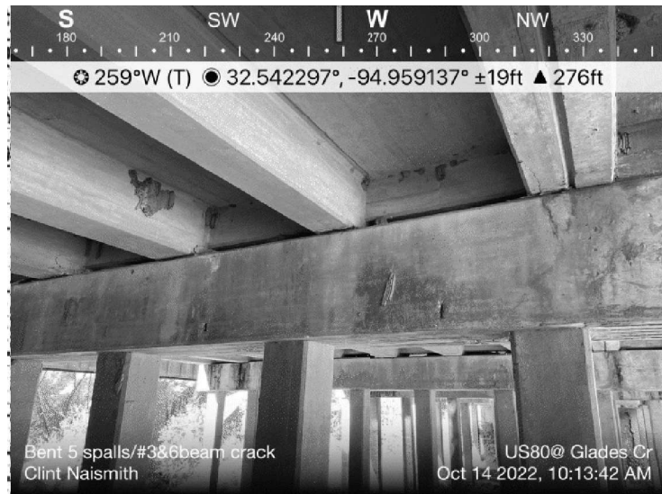
TYPICAL SPALL (SBI) PHOTOS
