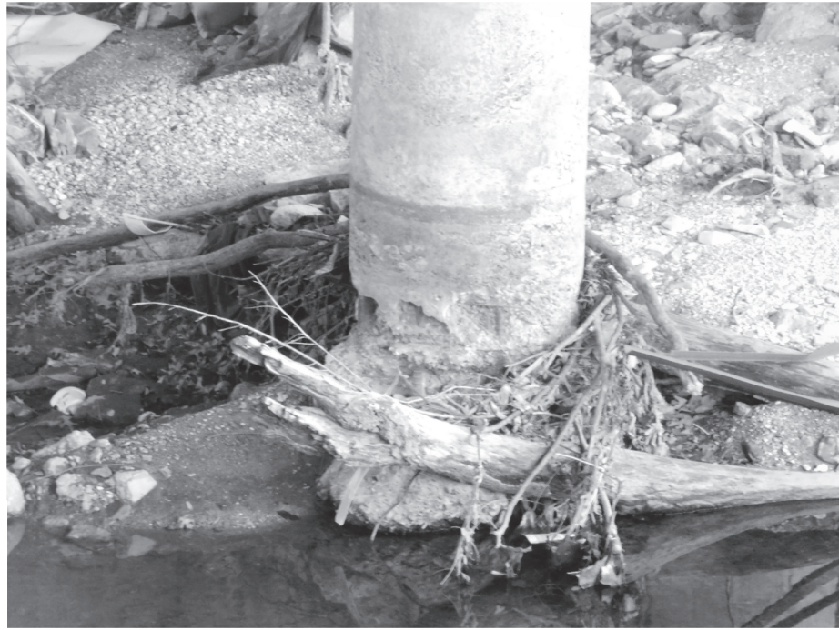
(A) CONCRETE REPAIR (VERTICAL & OVERHEAD)
