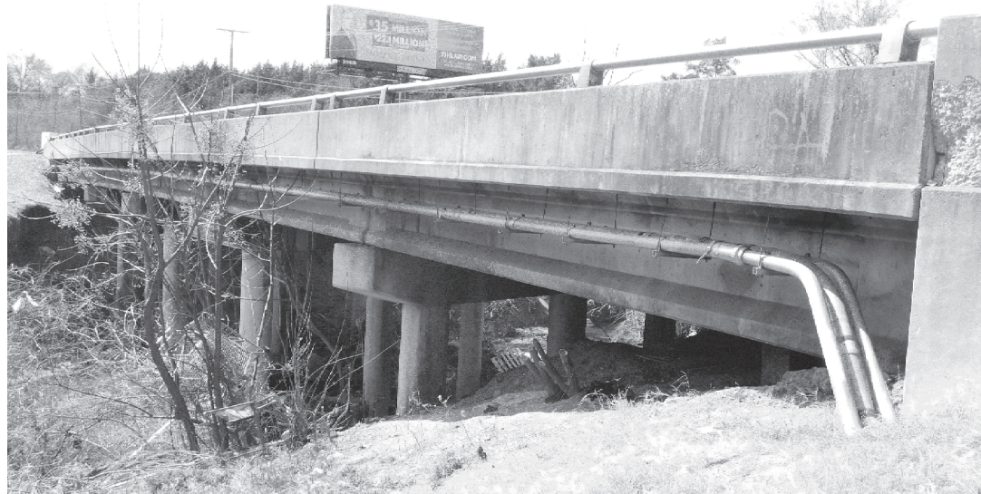
(C) RETROFIT RAIL (TY C221)(HPC)
