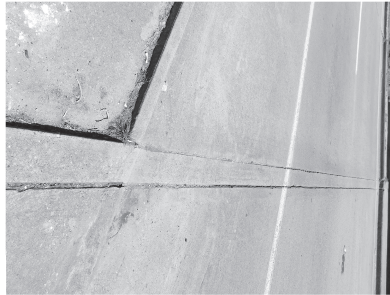
(B) CLEANING AND SEALING EXIST JOINTS(CL7)
