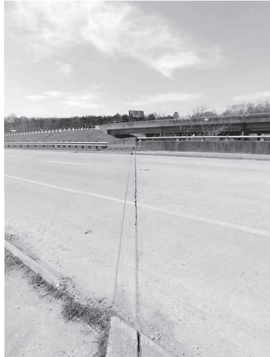
(B) CLEANING AND SEALING EXIST JOINTS(CL7)
