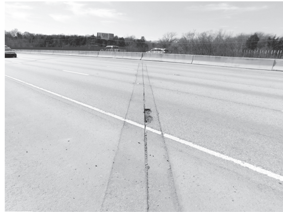
(B) CLEANING AND SEALING EXIST JOINTS(CL7)
