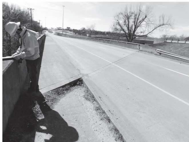
(E) SIDEWALK REMOVAL AND REPLACE
