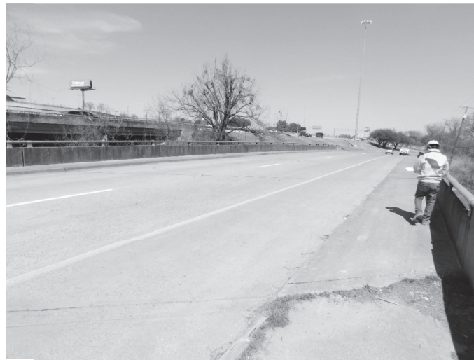
(C) RETROFIT RAIL (TY C221)(HPC)
