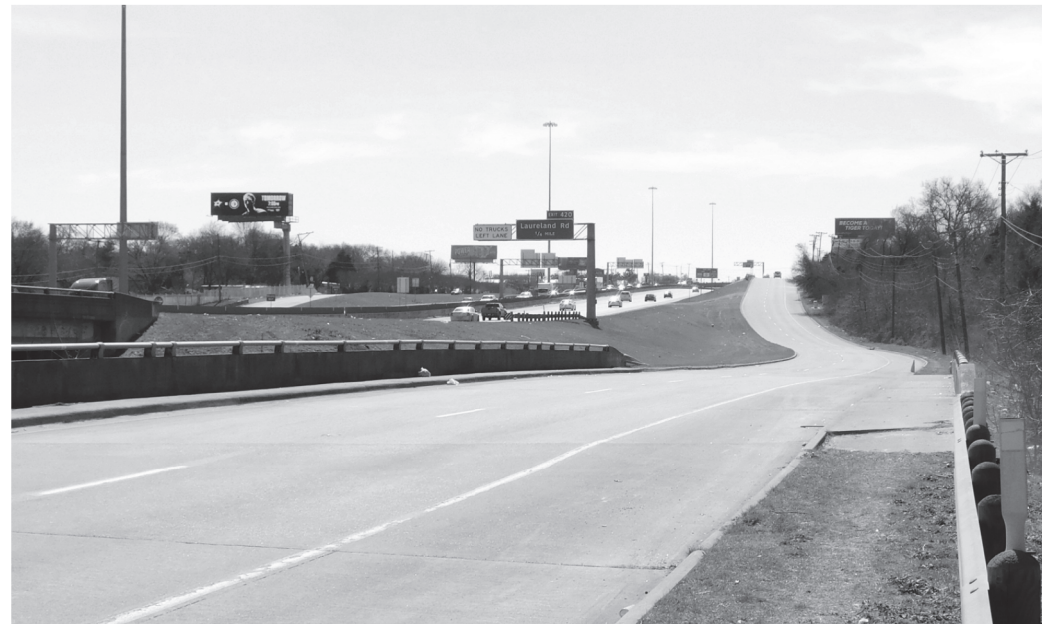
(E) SIDEWALK REMOVAL AND REPLACE
