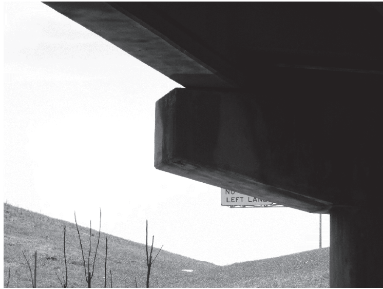
(A) CONCRETE REPAIR (VERTICAL & OVERHEAD)
