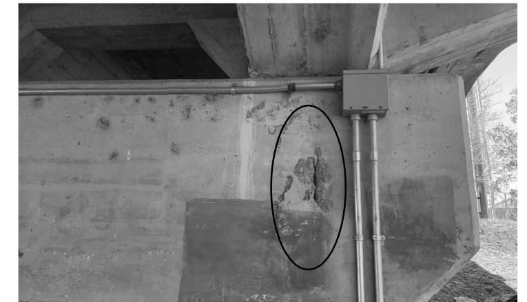
BENT CAP 1, SOUTH FACE
