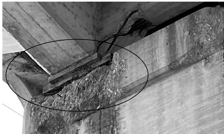
PIER CAP 3, NORTH FACE, GIRDER D
