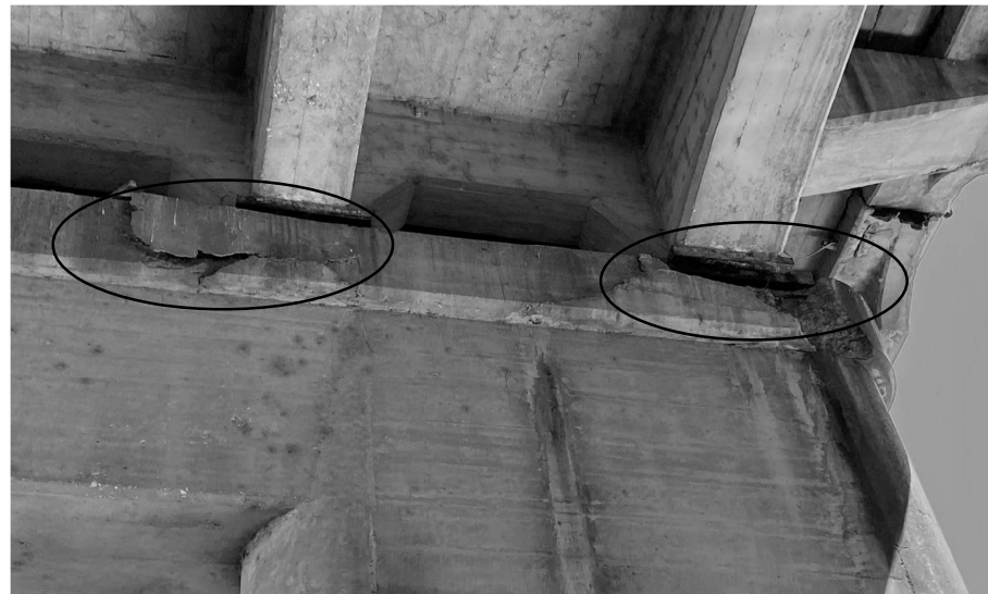
PIER CAP 3, NORTH FACE, GIRDERS A & B
