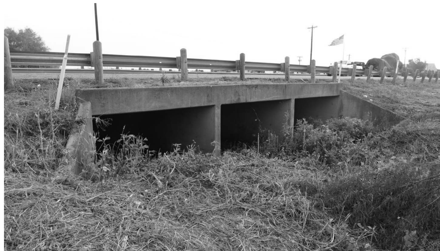
SOUTH BRIDGE ELEVATION - LOOKING NORTHEAST
