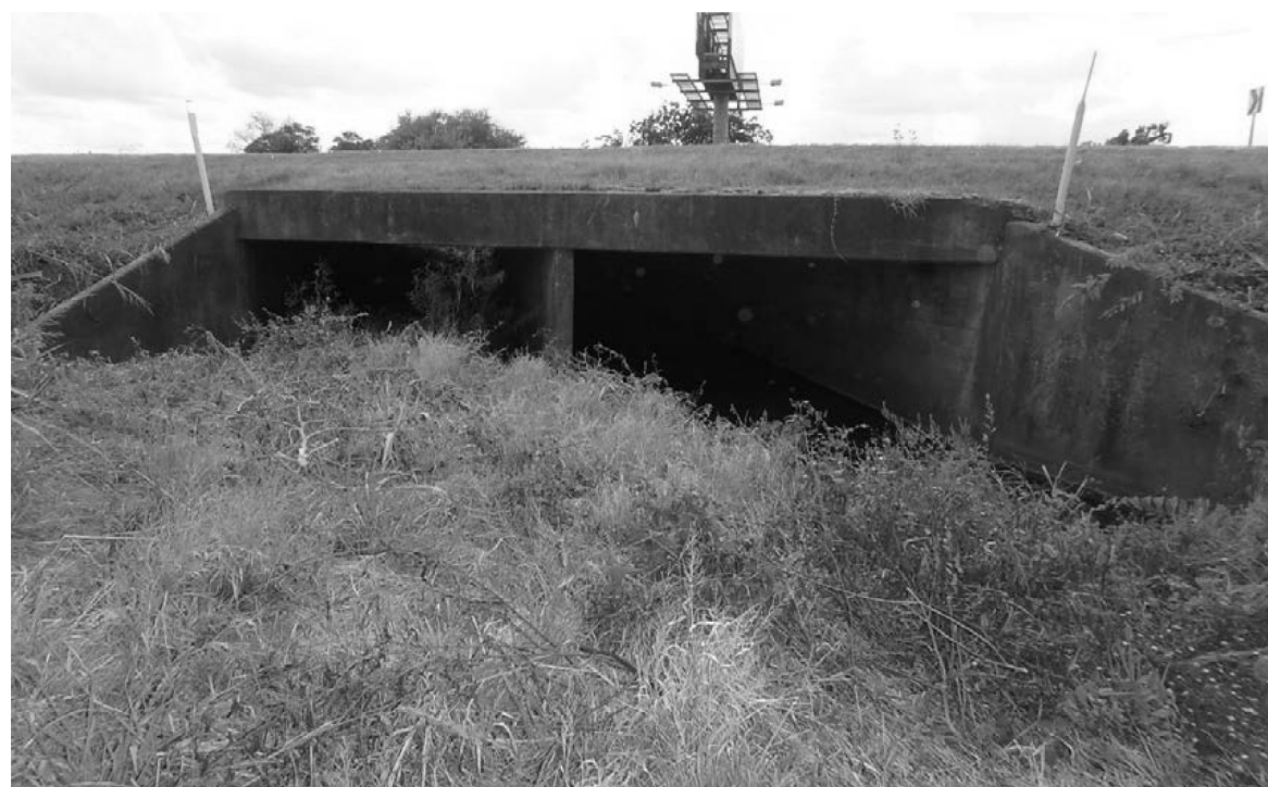
CHANNEL DOWNSTREAM THROUGH STRUCTURE (LOOKING SOUTH)
