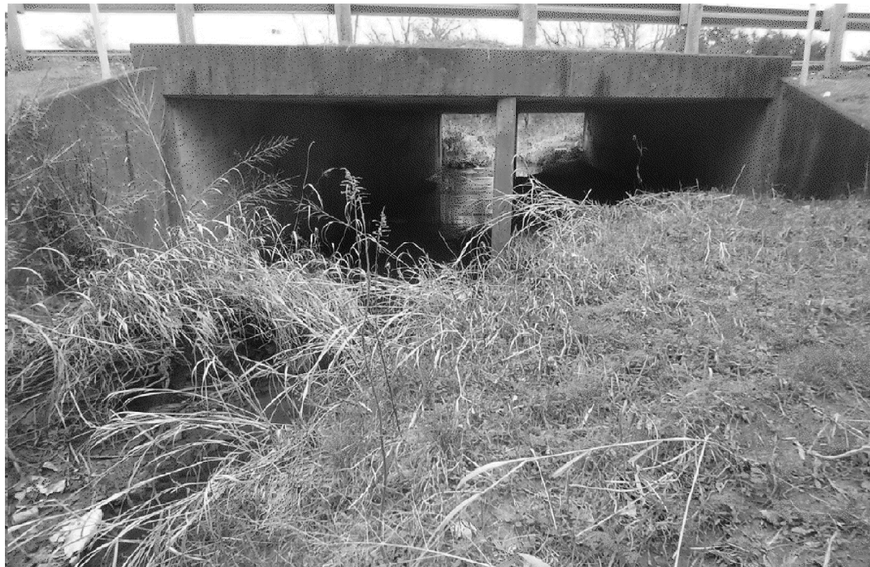
SOUTH SIDE OF CULVERT LOOKING NORTH
