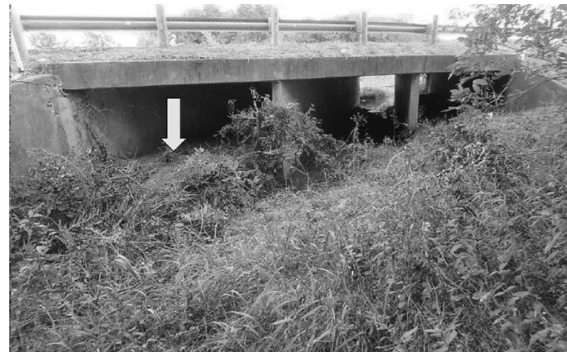
NORTH OF BRIDGE (CHANNEL US) LOOKING SOUTH
