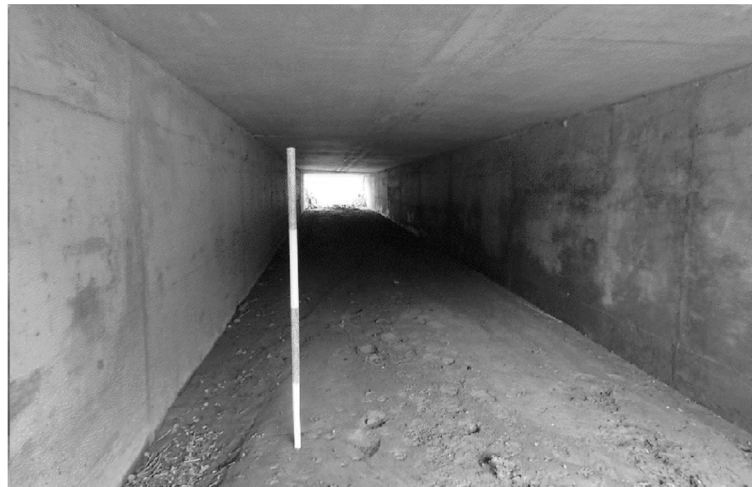
CULVERT CLEANING - AGGREGATION
