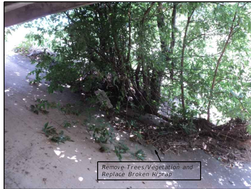
CONCRETE RIPRAP REPLACEMENT SHOWING LIMITS OF TREE REMOVAL/REPAIR
