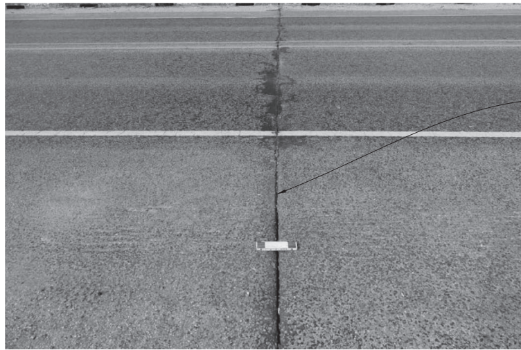
BRIDGE DECK JOINT OVER BENT #10
