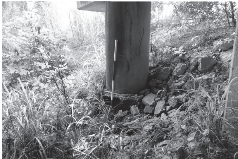
EXPOSED NE COLUMN DRILL SHAFT OF BENT #13
