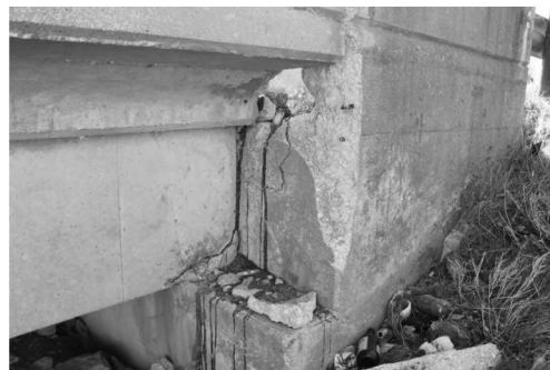
Backwall Spall
