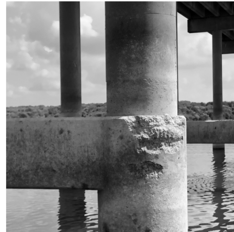
Concrete Spall
