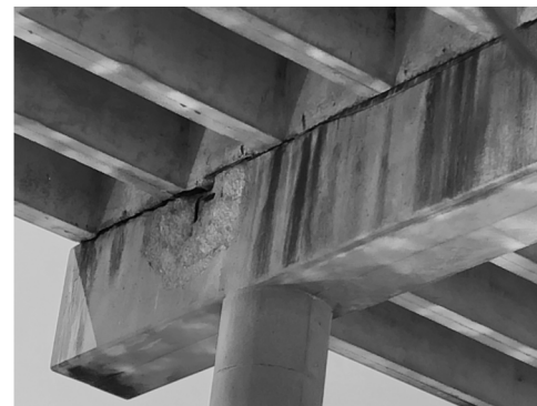
Concrete Spall
