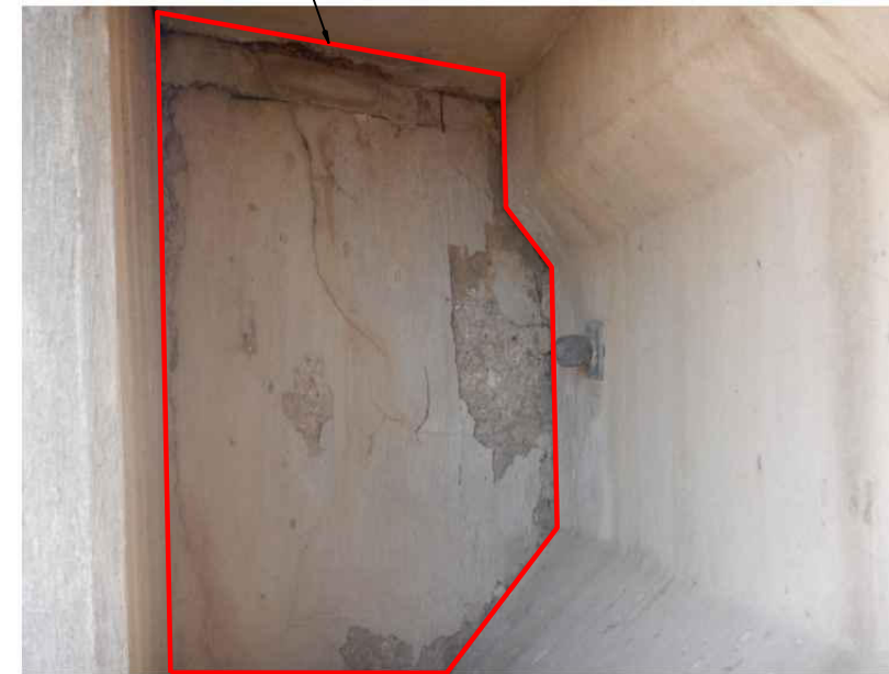
PHOTO 31 Showing Spall at Abutment #1 (West Corner of Backwall)
