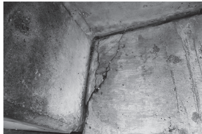
ABUTMENT 1 DETERIORATION
