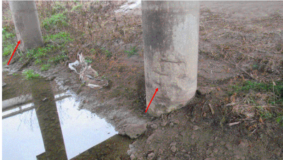
COLUMNS - LOOKING NORTHEAST VIEW 5782
