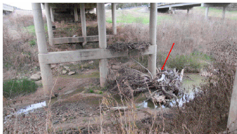
CHANNEL BED - LOOKING SOUTHEAST VIEW 6190
