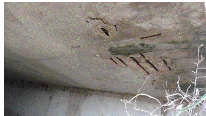
SOUTH BARREL - LOOKING SOUTHEAST VIEW 1586
