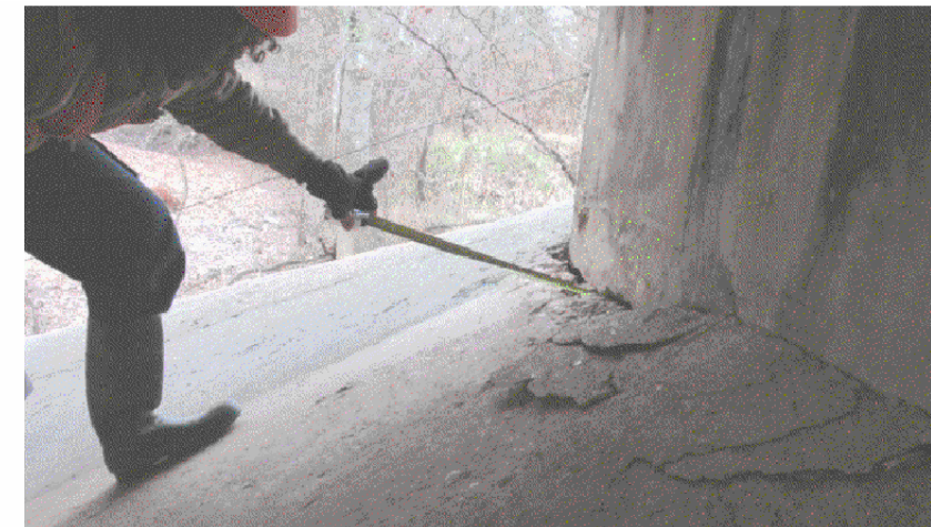
SOUTHWEST RIPRAP - LOOKING SOUTHEAST VIEW 1441
