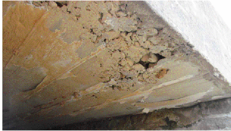
CENTER SPAN SOFFIT - LOOKING NORTHWEST VIEW 771
