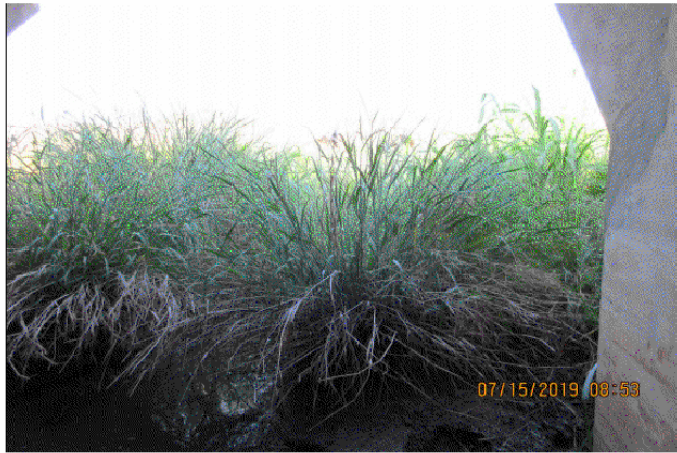
BUILDUP UPSTREAM SIDE Looking SW IMG. 0050
