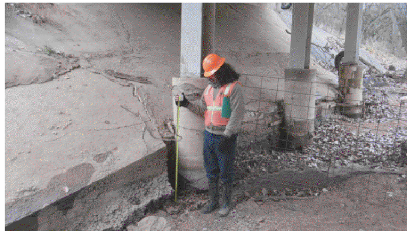
NORTHEAST INTERIOR BENT - LOOKING EAST VIEW 1439
