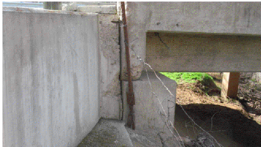
SOUTHEAST WINGWALL - LOOKING WEST VIEW 1776
