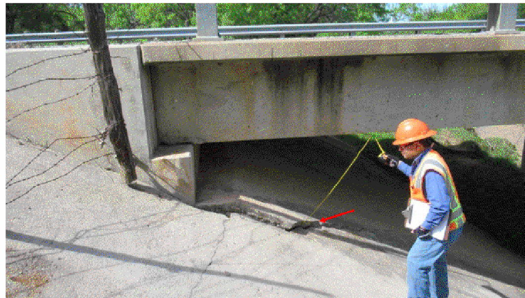
SOUTHWEST EMBANKMENT RIPRAP - LOOKING NORTH VIEW 2150
