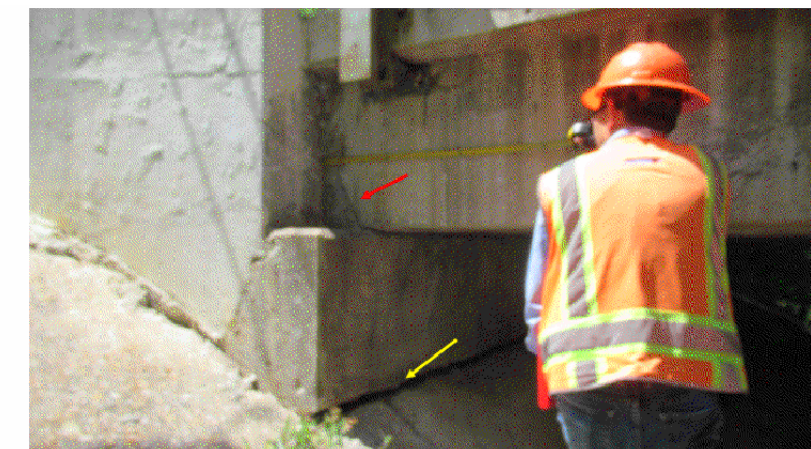
SOUTH EXTERIOR PAN GIRDER - LOOKING NORTHWEST VIEW 8430
