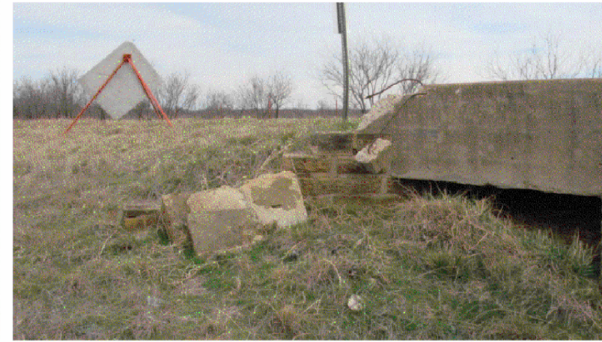
NORTHWEST WINGWALL - LOOKING NORTHEAST VIEW 773
