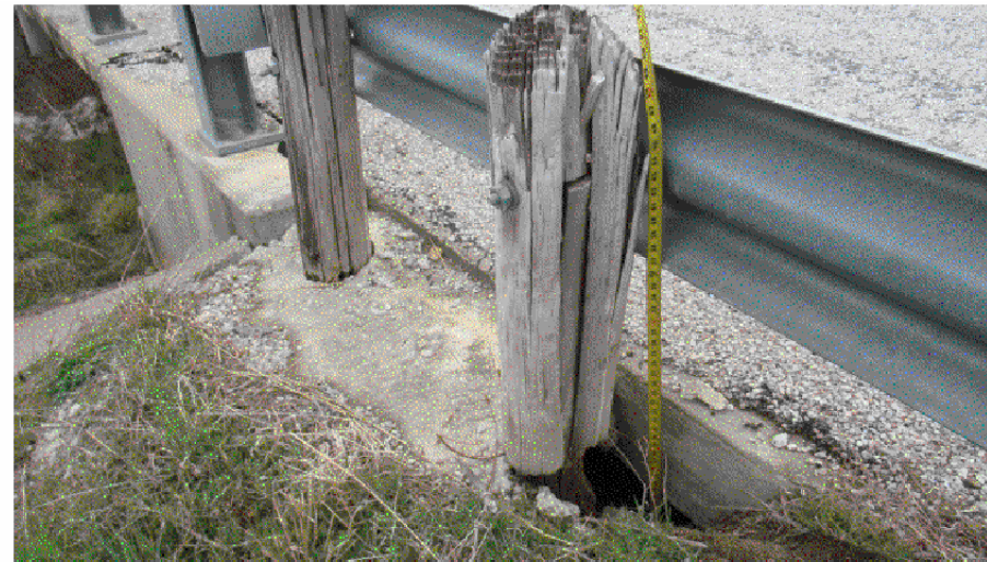
NORTHWEST EMBANKMENT - LOOKING SOUTHEAST VIEW 6180
