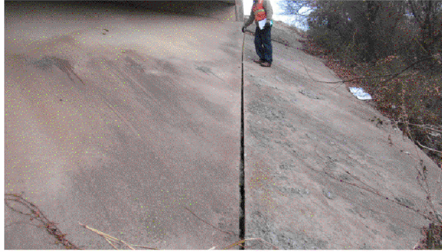
NORTHEAST EMBANKMENT RIPRAP - LOOKING NORTH VIEW 854
