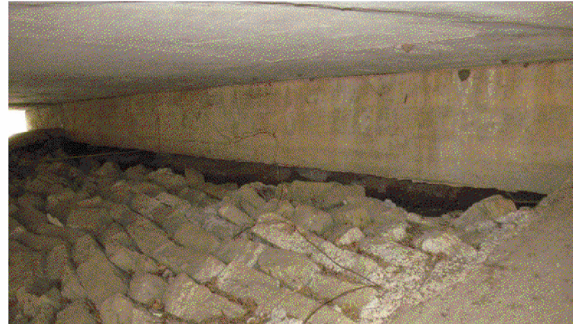
SOUTH ABUTMENT CAP - LOOKING SOUTHEAST VIEW 6297
