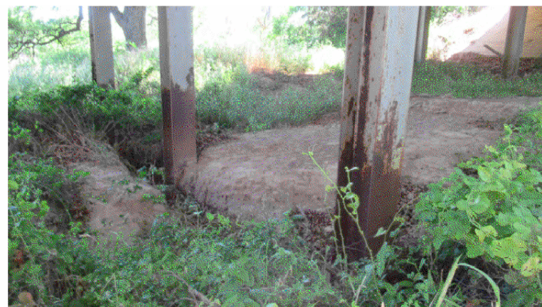
STEEL PILES AT BENT 6 - LOOKING SOUTHWEST VIEW 8434
