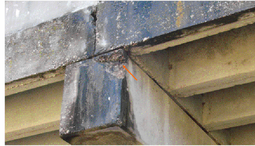
BENT CAP 3 - LOOKING SOUTHEAST
