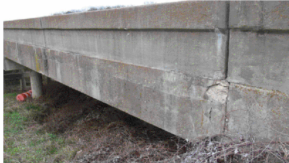
NORTH EXTERIOR BEAM - LOOKING SOUTHEAST VIEW 6248
