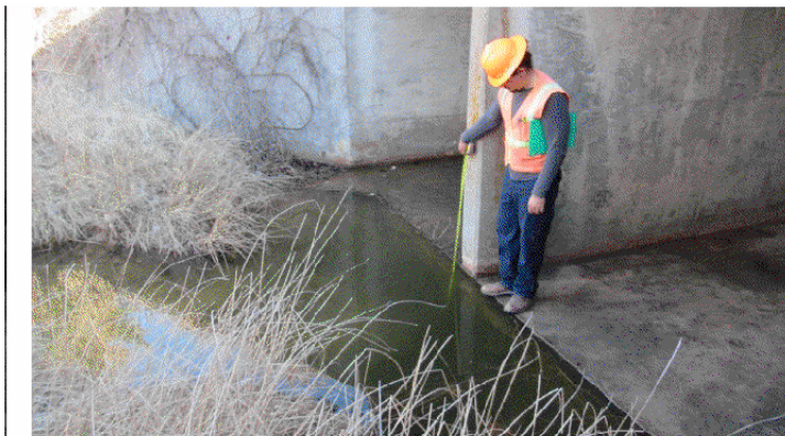
UPSTREAM TOEWALL - LOOKING SOUTHEAST
