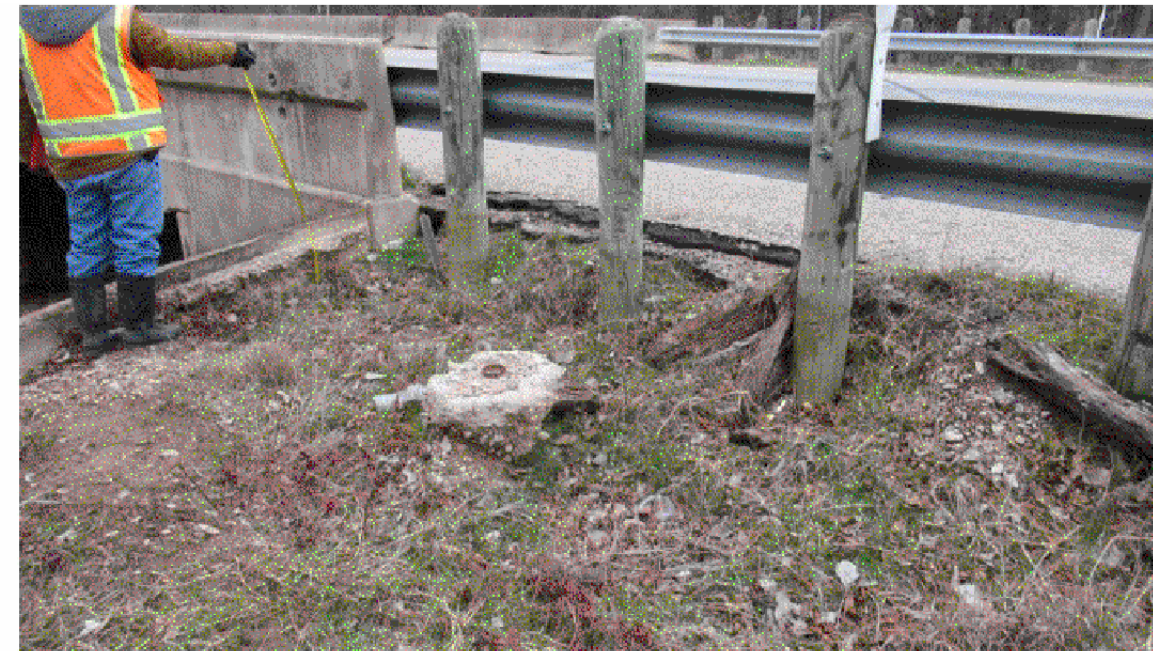
SOUTHWEST EMBANKMENT - LOOKING NORTHEAST VIEW 6299
