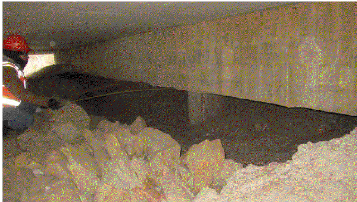
NORTH ABUTMENT CAP - LOOKING NORTHWEST VIEW 6295
