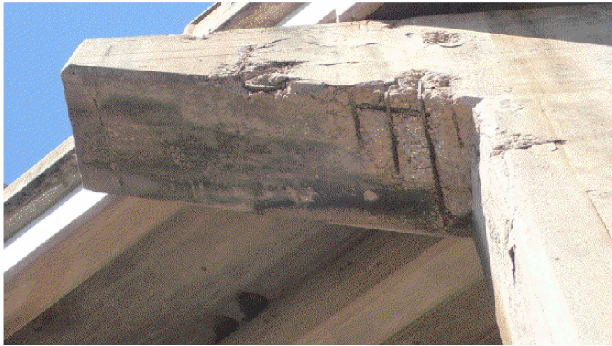
BENT 4 CAP - LOOKING NORTHWEST VIEW 396
