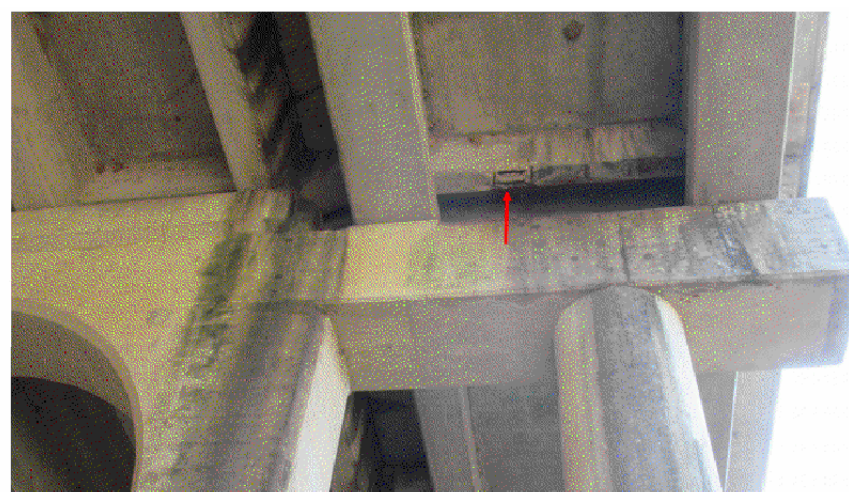
NORTHWEST DIAPHRAGM - LOOKING SOUTHWEST VIEW 6904
