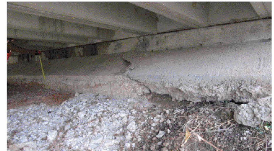
EAST ABUTMENT - LOOKING NORTHEAST VIEW 6150
