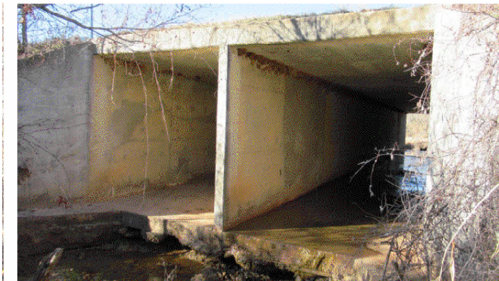
ELEVATION VIEW - LOOKING NORTHWEST
