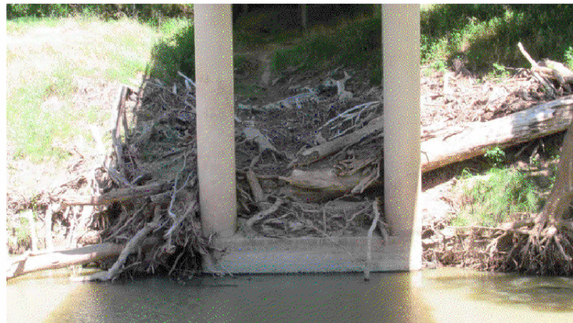
EAST CHANNEL BANK - LOOKING EAST VIEW 8435
