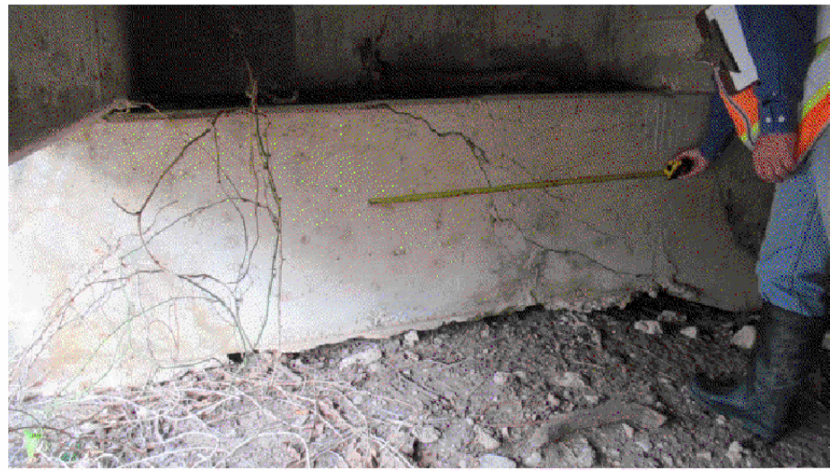
NORTHWEST ABUTMENT CAP - LOOKING NORTHWEST VIEW 6963
