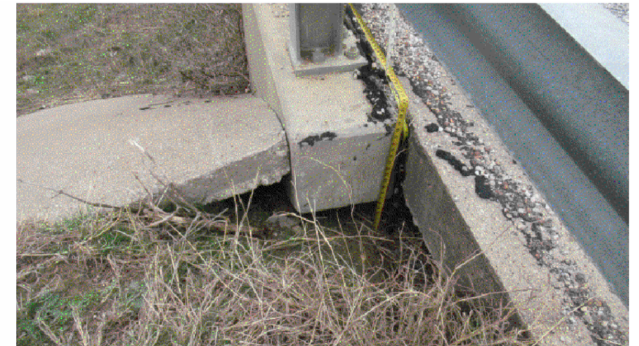
SOUTHEAST EMBANKMENT - LOOKING NORTH WEST VIEW 6176
