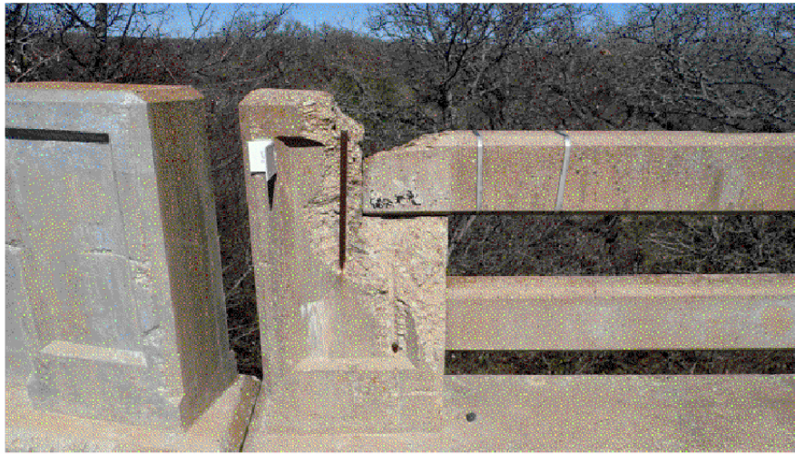
NORTH RAIL AT SPAN 1 - LOOKING NORTH VIEW 367
