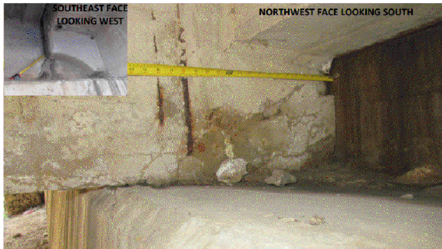
BEAM 8 - LOOKING SOUTH VIEW 6918 & 6912
