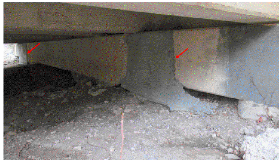
SOUTHEAST ABUTMENT CAP - LOOKING NORTHEAST VIEW 6971
