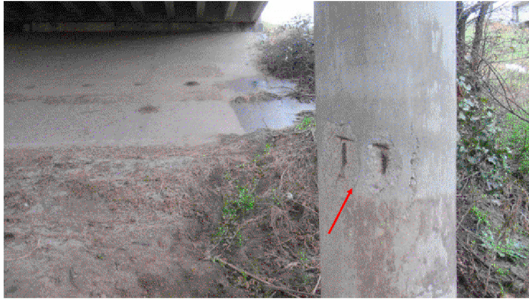
NORTH EXTERIOR COLUMN - LOOKING WEST VIEW 5790
