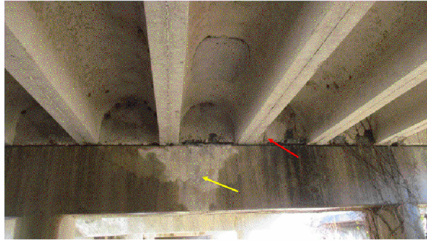
WEST INTERIOR BENT CAP - LOOKING EAST
