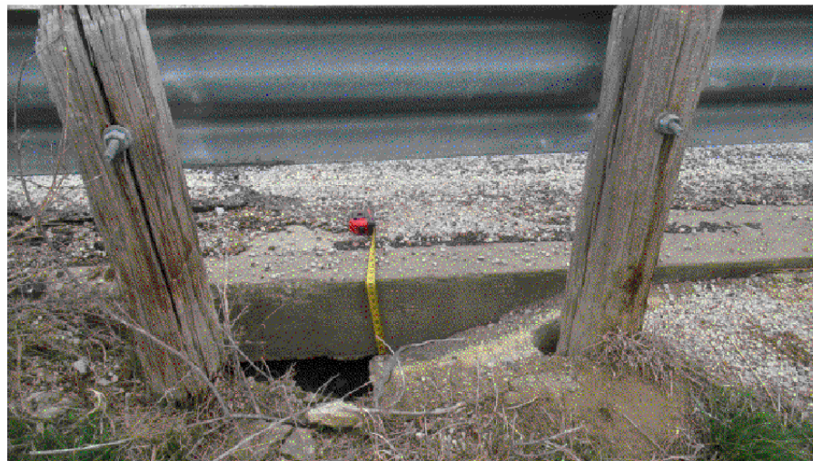
SOUTHWEST EMBANKMENT - LOOKING NORTH VIEW 6182
