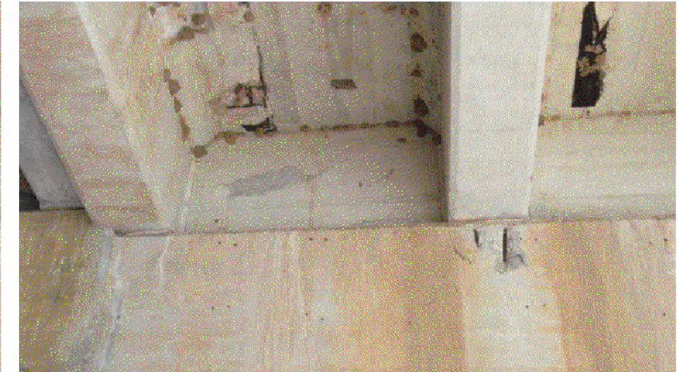
INTERIOR BENT CAP - LOOKING SOUTH VIEW 1774
