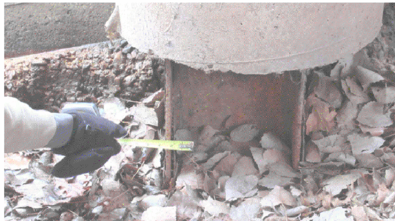
NORTHEAST INTERIOR BENT - LOOKING NORTHEAST VIEW 1440
