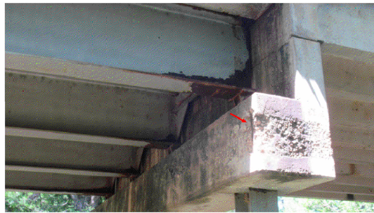
BENT 3 - LOOKING NORTHEAST VIEW 8423
