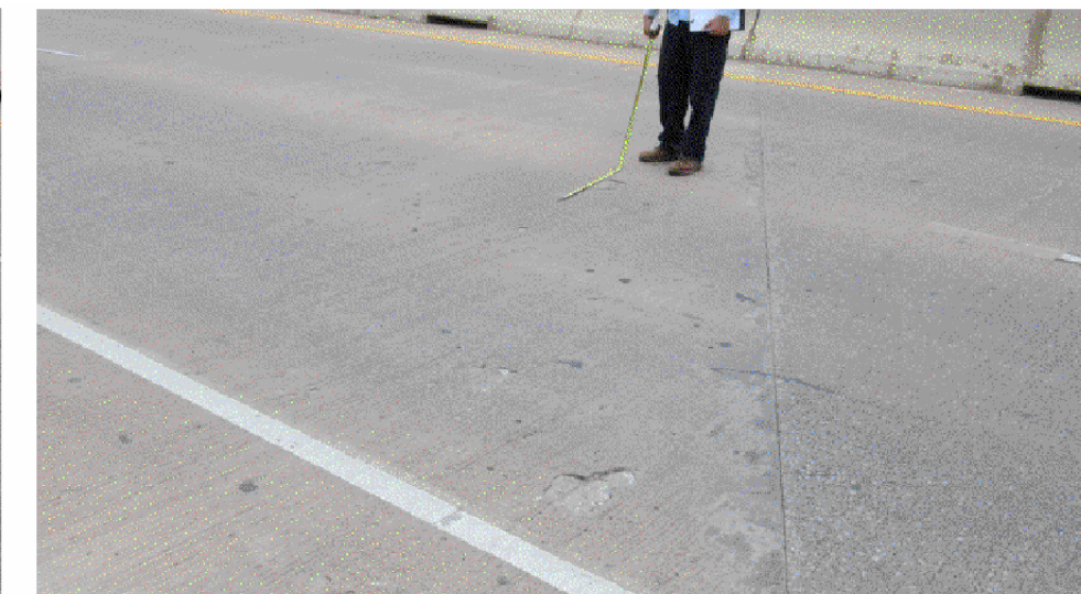
SPAN 5 DECK - LOOKING SOUTHWEST VIEW 2094
