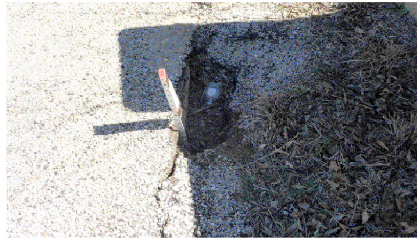
SW APPROACH CORNER - LOOKING EAST VIEW 366
