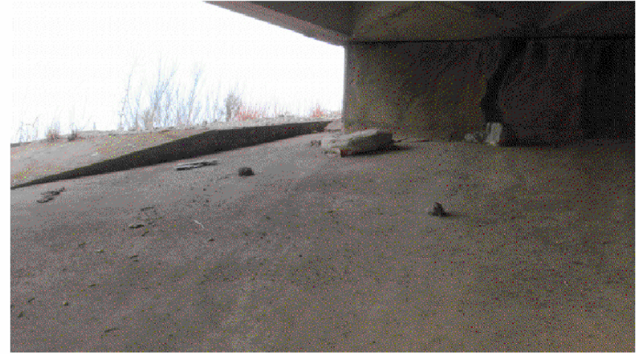
NORTHWEST EMBANKMENT RIPRAP - LOOKING NORTHWEST VIEW 852
