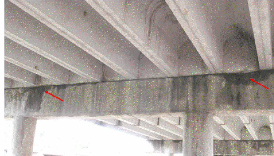
BENT CAP 3 - LOOKING NORTHEAST VIEW 6227
