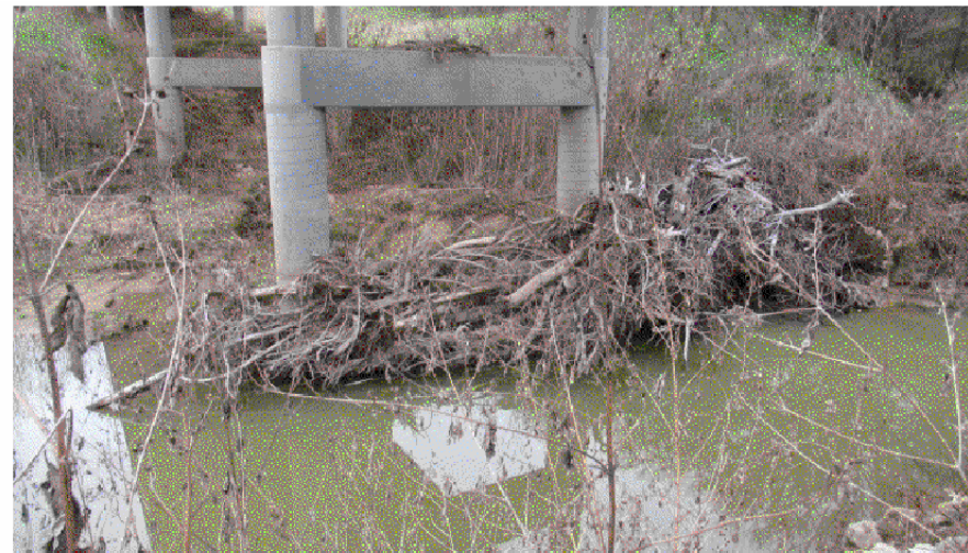
CHANNEL BED - LOOKING SOUTHEAST VIEW 6185
