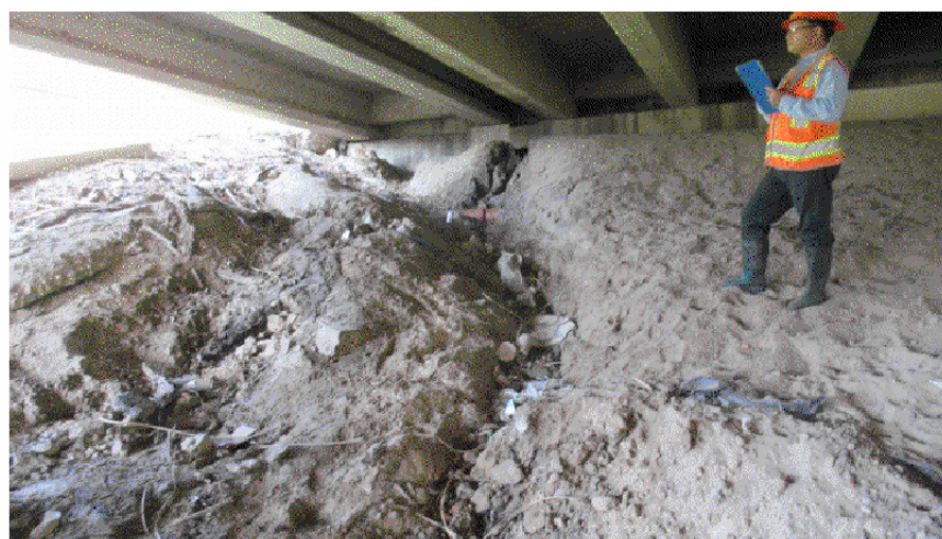
NORTHEAST CHANNEL BANK - LOOKING NORTHEAST VIEW 6893
