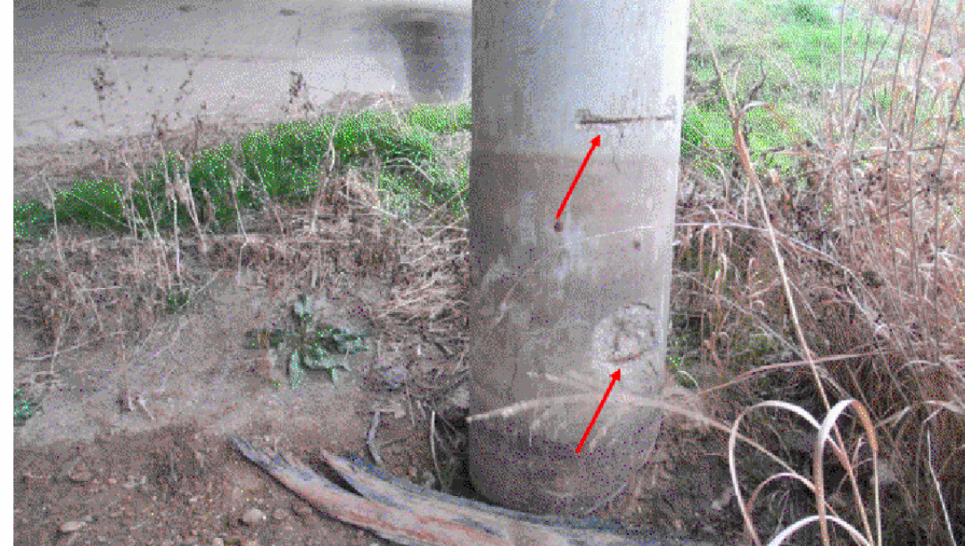
SOUTH EXTERIOR COLUMN - LOOKING SOUTHEAST VIEW 5783
