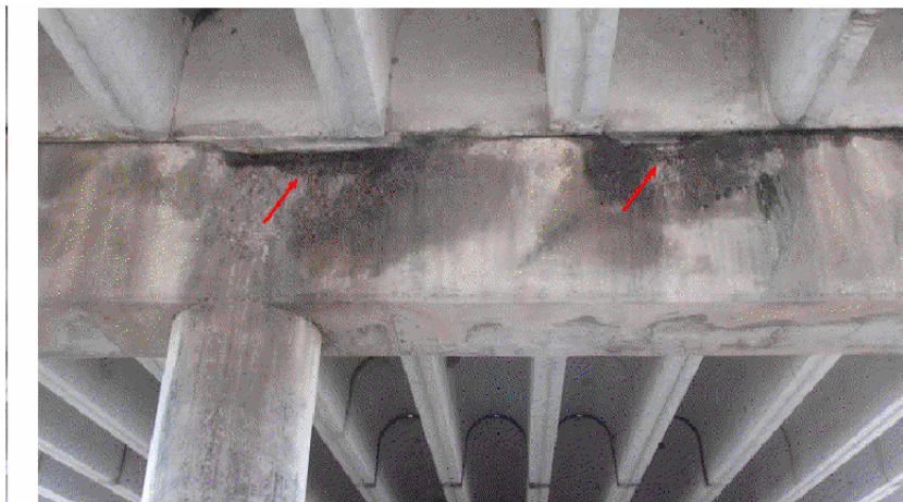
BENT CAP 2 - LOOKING WEST VIEW 6188
