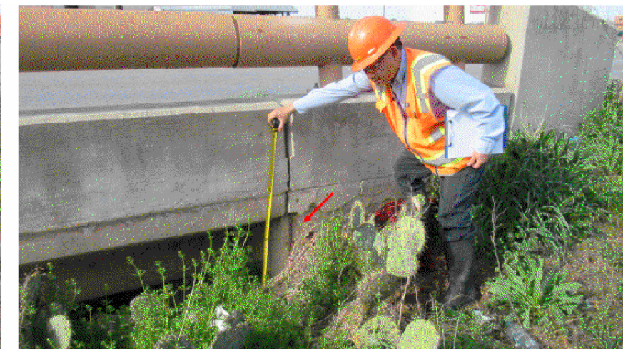
EAST WINGWALL - LOOKING NORTH VIEW 6885
