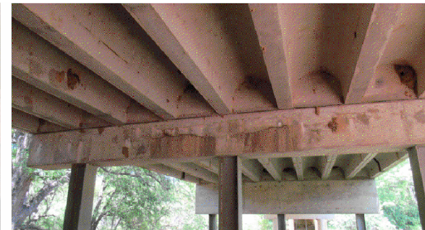
BENT CAP 7 - LOOKING EAST VIEW 8431
