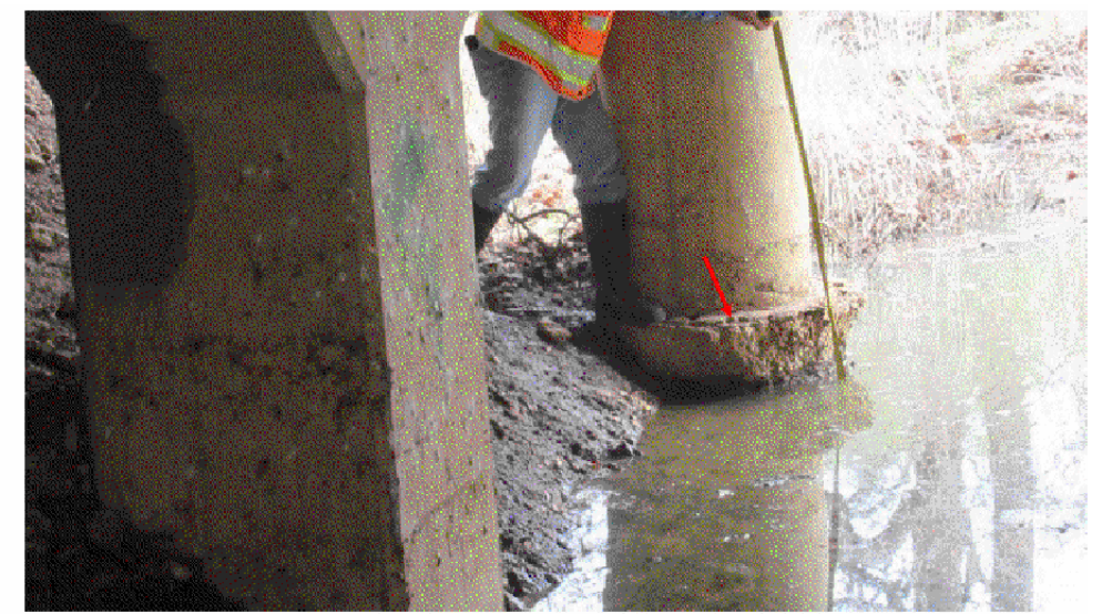
DRILLED SHAFT - LOOKING NORTH VIEW 6966
