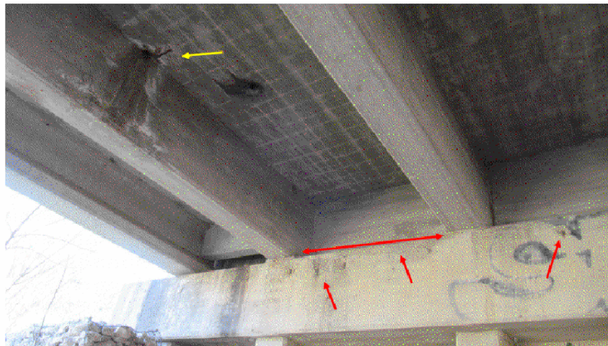
SOUTHWEST ABUTMENT CAP - LOOKING SOUTHWEST VIEW 6907
