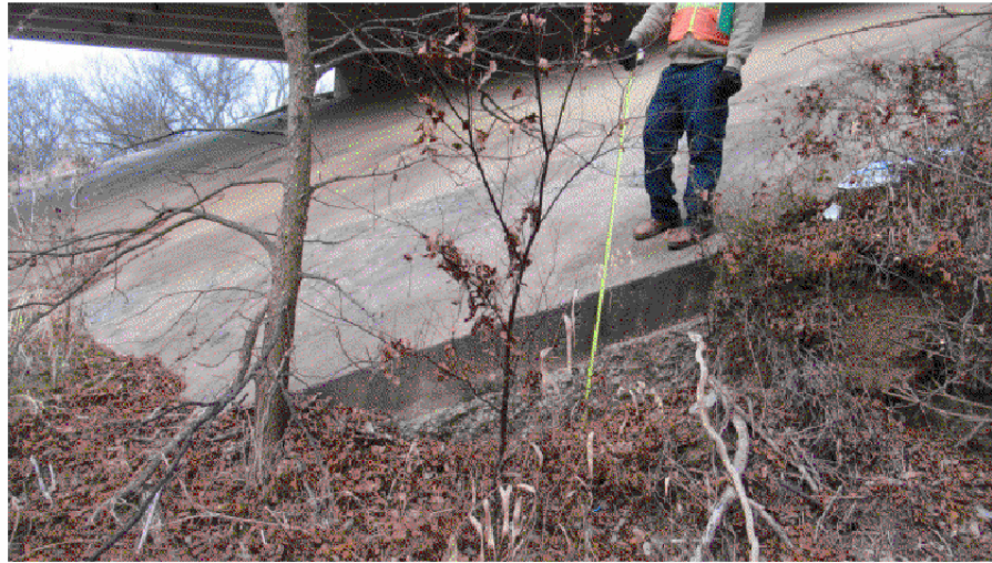
NORTHEAST EMBANKMENT RIPRAP - LOOKING NORTHWEST VIEW 853
