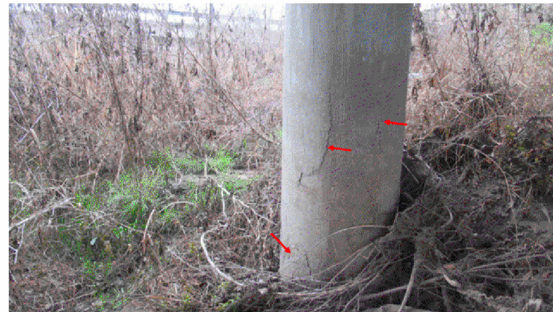
SOUTH EXTERIOR COLUMN - LOOKING SOUTHWEST VIEW 5791
