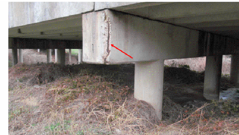
BENT CAP 7 - LOOKING NORTHWEST VIEW 6197
