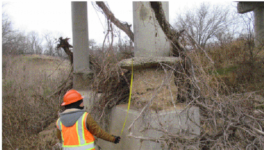
DRILLED SHAFTS - LOOKING SOUTHWEST VIEW 6184
