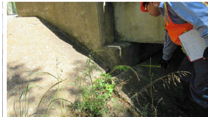
EAST ABUTMENT RIPRAP - LOOKING SOUTHEAST VIEW 8428
