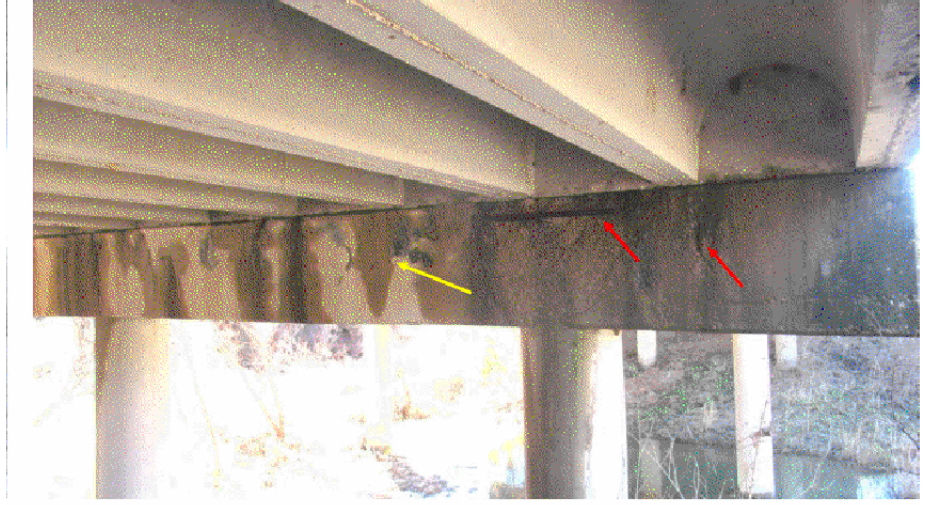
EAST INTERIOR BENT CAP - LOOKING WEST
