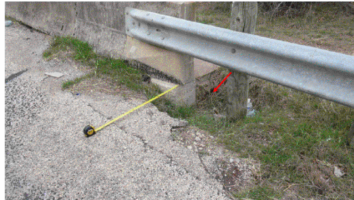
SOUTHEAST BRIDGE CORNER - LOOKING NORTHEAST VIEW 6290
