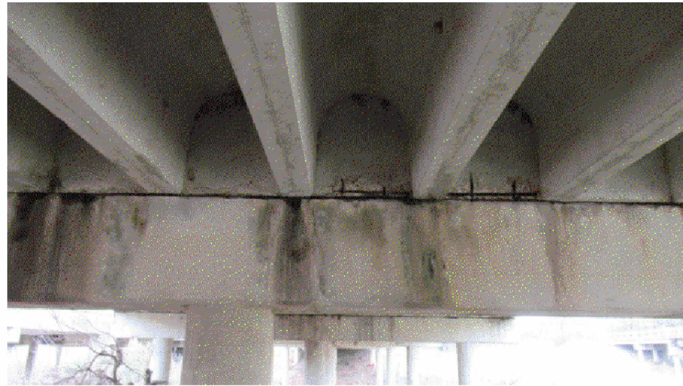
DIAPHRAGMS - LOOKING WEST VIEW 6221
