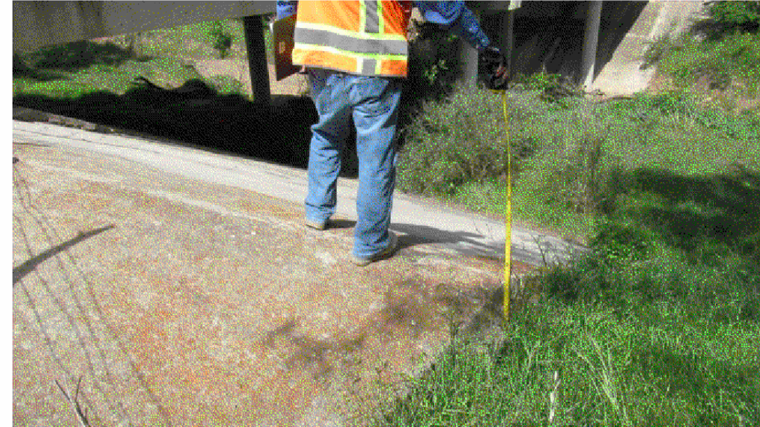
SOUTHWEST EMBANKMENT RIPRAP - LOOKING EAST VIEW 2149
