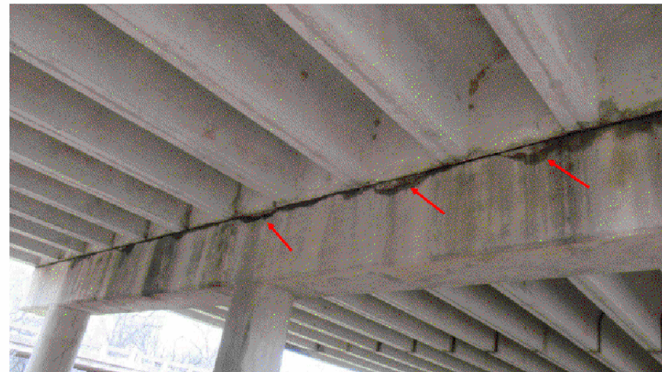
BENT CAP 6 - LOOKING NORTHEAST VIEW 6222
