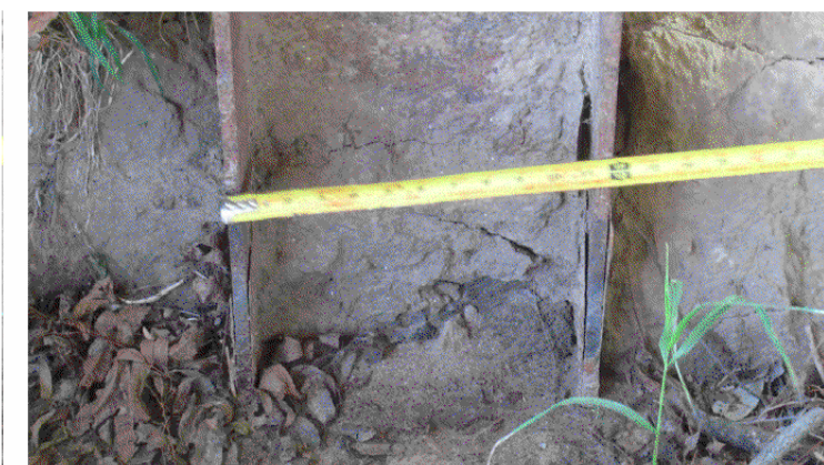
CENTER PILE AT BENT 6 - LOOKING EAST VIEW 8437
