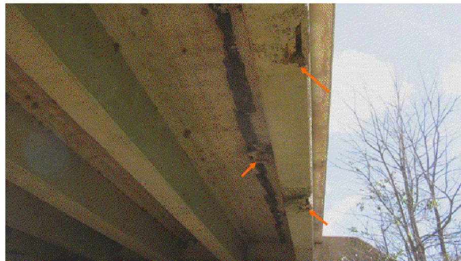
WEST EXTERIOR BEAM - LOOKING SOUTHEAST VIEW 1772
