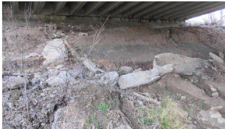
WEST ABUTMENT - LOOKING NORTHWEST VIEW 6158
