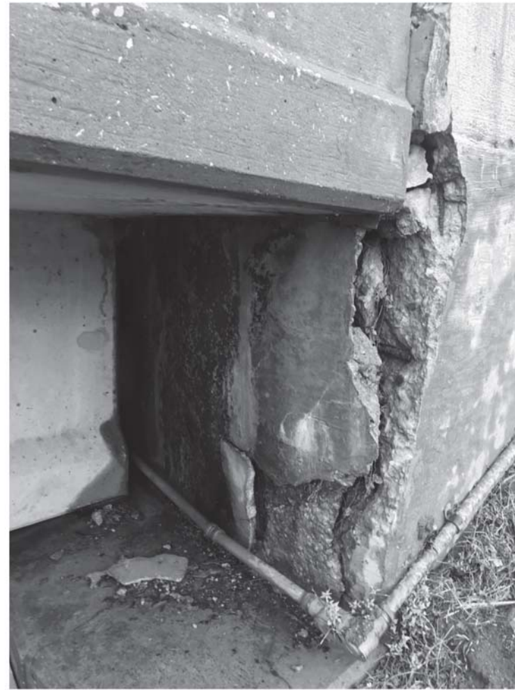
TYPICAL BACKWALL/WINGWALL REPAIR AT STRUCTURES -084 AND -085
