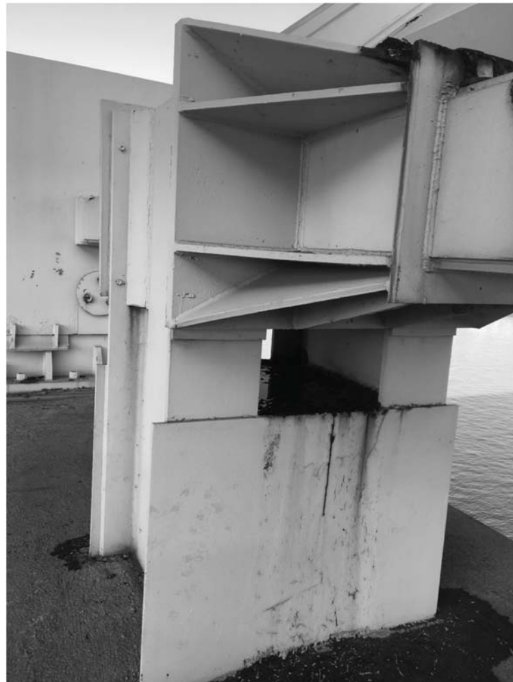
PHOTO OF BOTTOM OF WINDSHOE (TYP.)
