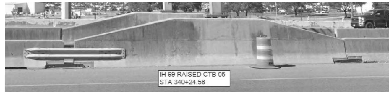
IH 69 RAISED CTB STA 340+24.58
