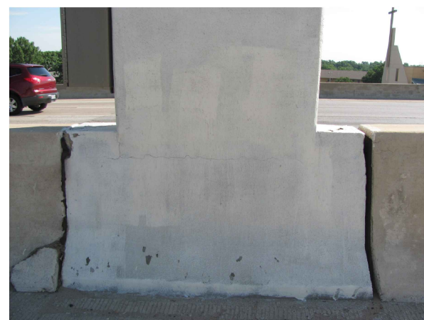
LOCATION OF CONC. CRACK REPAIR (ROUT AND SEAL) ON SOUTH FACE OF PARAPET FOUNDATION:
