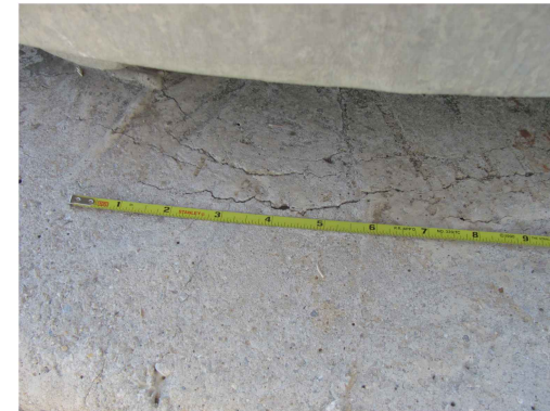
LOCATION OF CONC. CRACK REPAIR (GRAVITY) ON FOUNDATION TOP:
