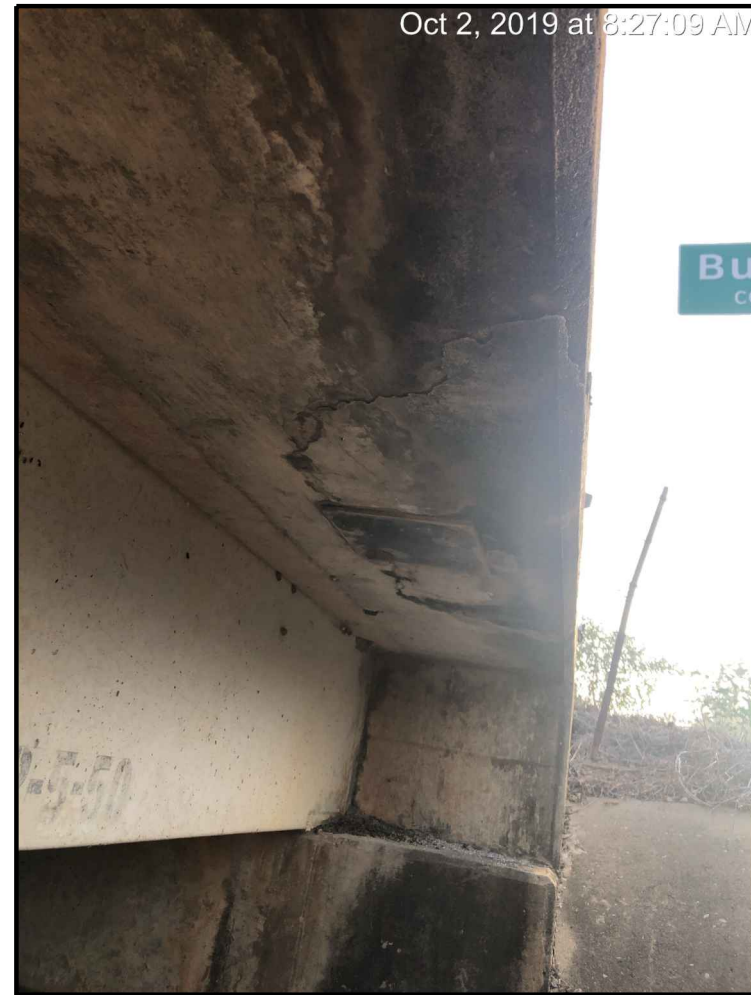
BRIDGE DECK SPALL AT SPAN NO. 17
