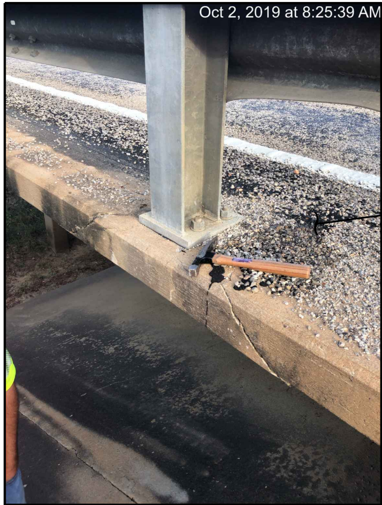
BRIDGE DECK SPALL AT SPAN NO. 17
