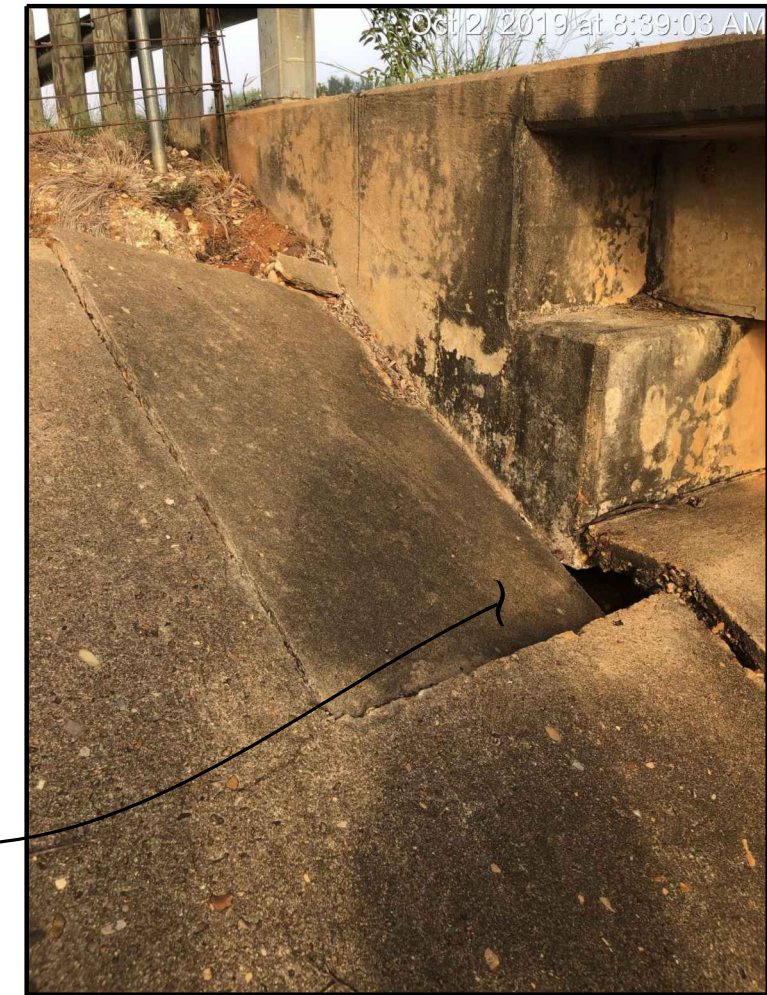
RIPRAP SETTLEMENT AT ABUTMENT NO. 1
