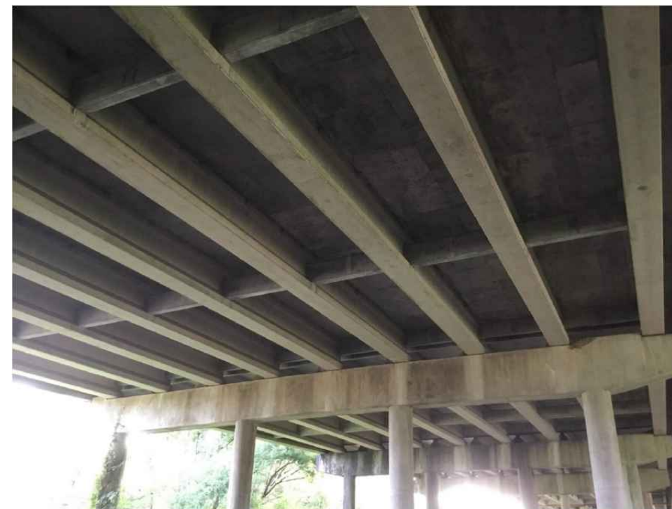
Typical bent cap photo.
