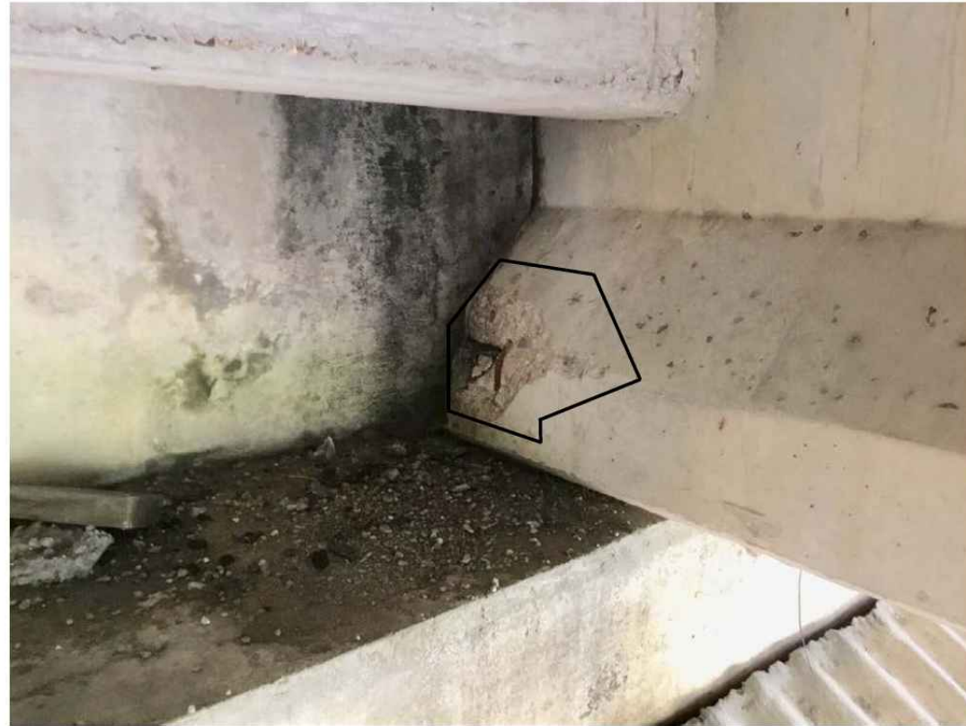
IH-610 Eastbound, Span 12R (East Endspan), Beam 2 from South at Abutment
