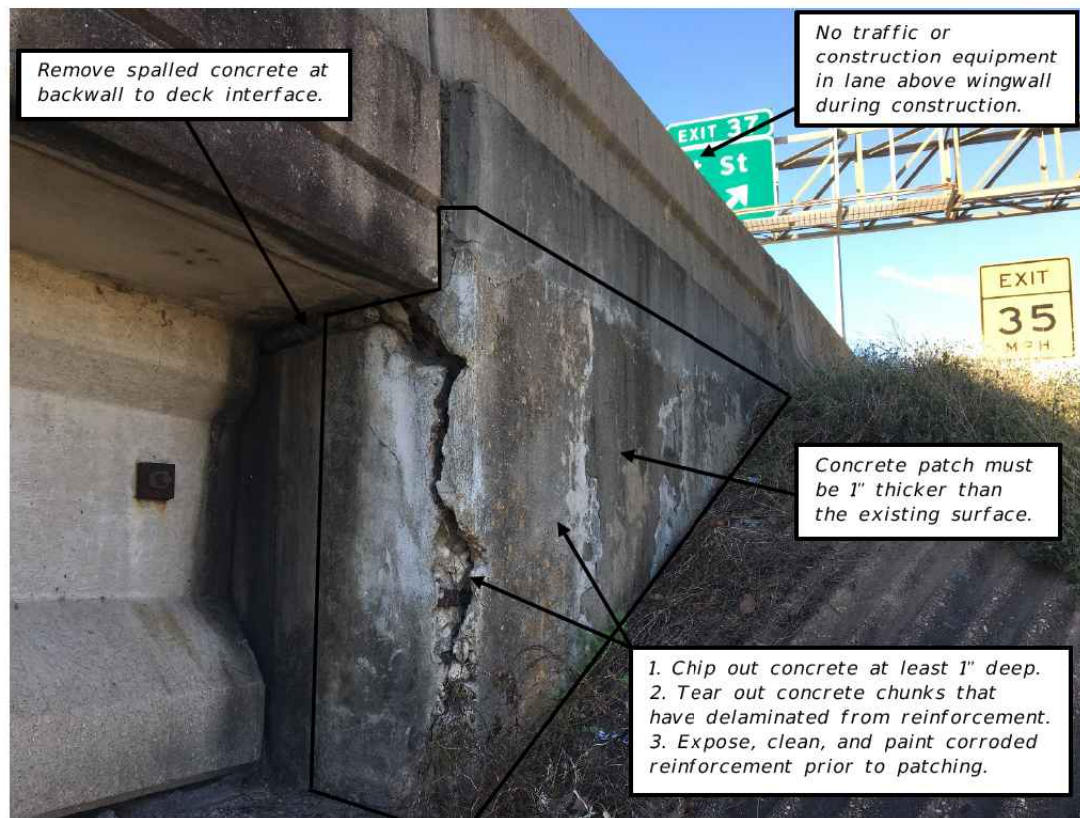
IH-610 Westbound, North-West Wingwall
