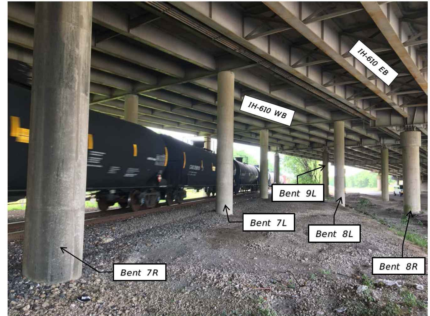
Overall View Looking North-East Under Bridge
