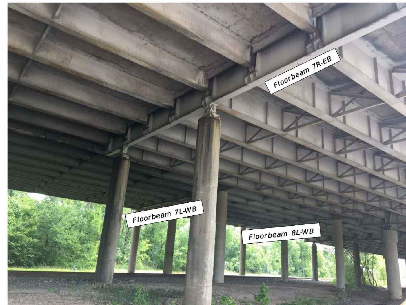
Floorbeam 7R-EB Looking North-East Under Bridge
