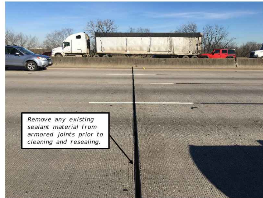
IH 610 Eastbound, Armored Joint at Bent 7R (picture of armored joint)
