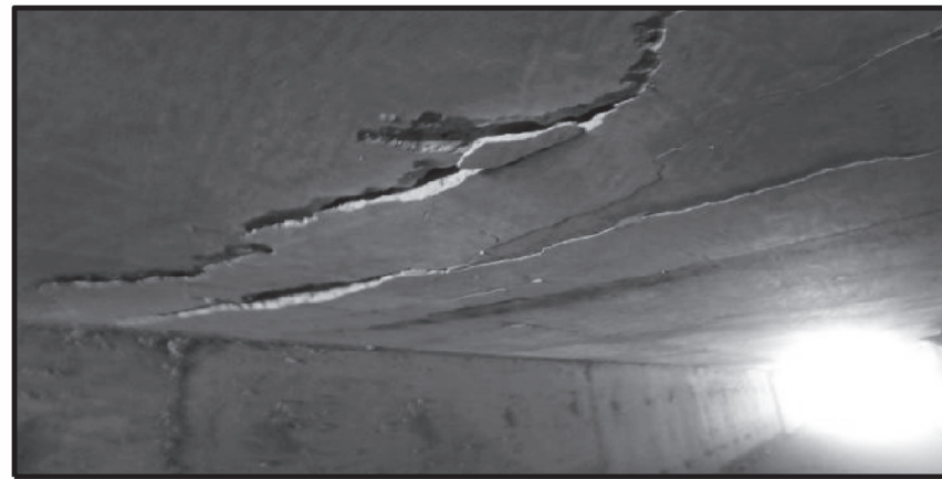
Repair Heavy Delamination in Soffit of Top Slab in Barrel 4 from W. Roughly 35 FT from South Opening
