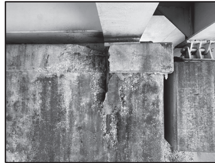
Spall at corner at Pier 7, Span 6. Looking West
