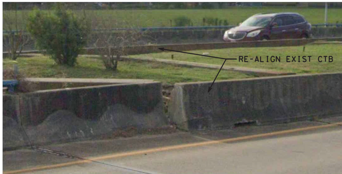
PHOTO OF EXISTING CONDITION LOOKING EAST FROM SOUTHBOUND LANES
