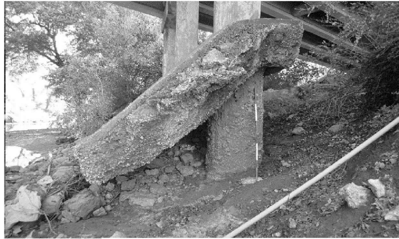
REMOVE CONCRETE RIPRAP AND PLACE ROCK RIPRAP AT BENT 4. (LOOKING EAST)
