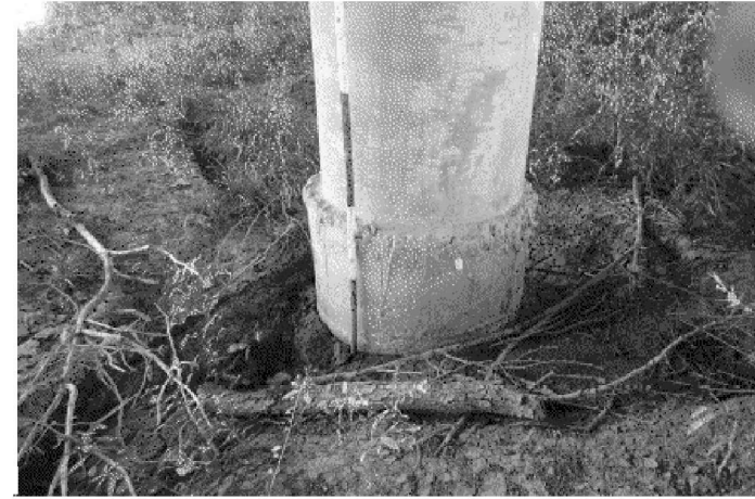
PLACE ROCK RIPRAP AT BENT 2. (LOOKING SOUTH)
