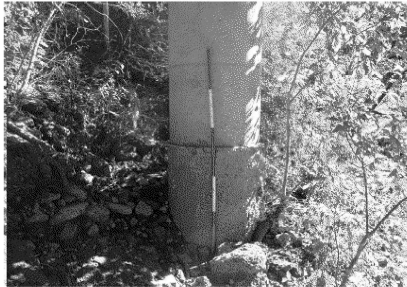
PLACE ROCK RIPRAP AT BENT 5. (LOOKING EAST)
