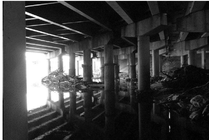
CLEAR DEBRIS AT BENT 6 AT NBML BRIDGE (LOOKING SOUTHEAST)
