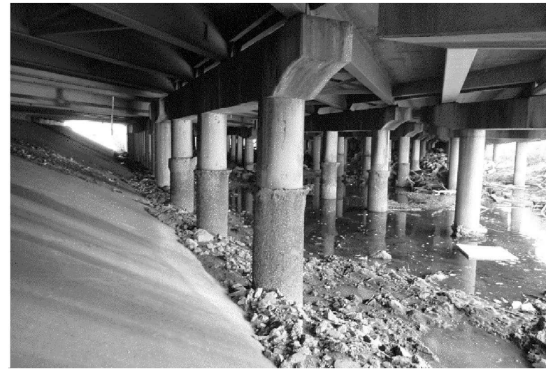
PLACE ROCK RIPRAP AT BENT 6, 7 AND 8 AT NBML BRIDGE (LOOKING NORTHWEST)
