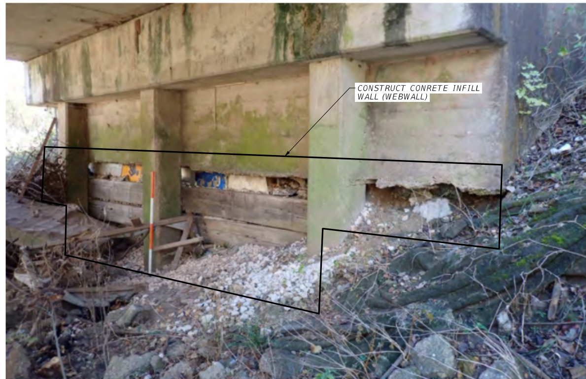
PHOTO 2 (SHOWING ABUTMENT NO. 3 ELEVATION)
