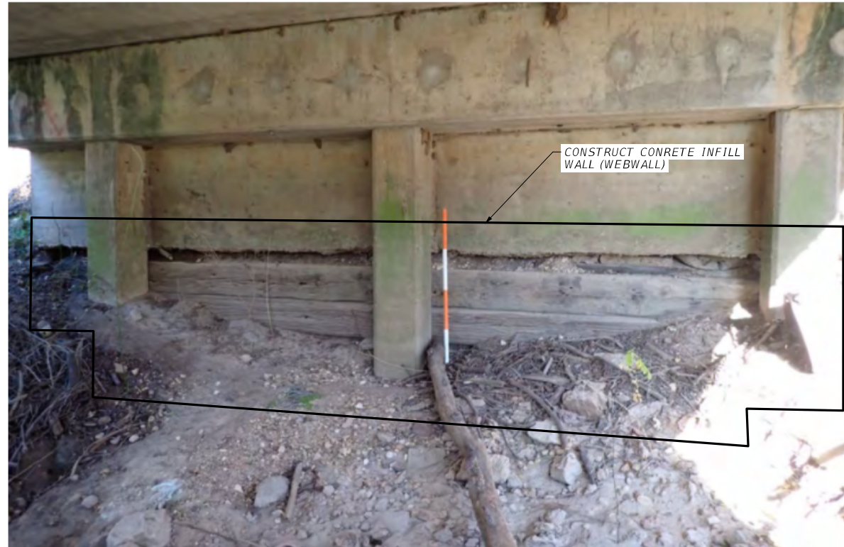
PHOTO 1 (SHOWING ABUTMENT NO. 1 ELEVATION)
