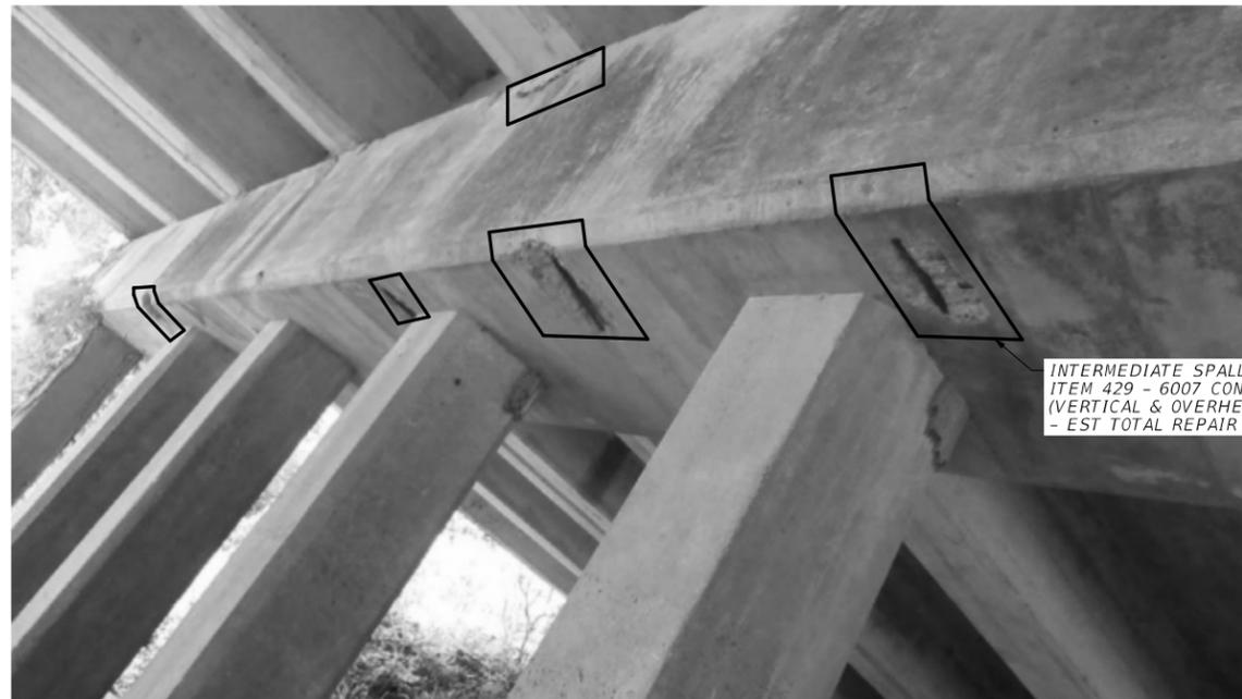
INTERMEDIATE SPALL REPAIR.
