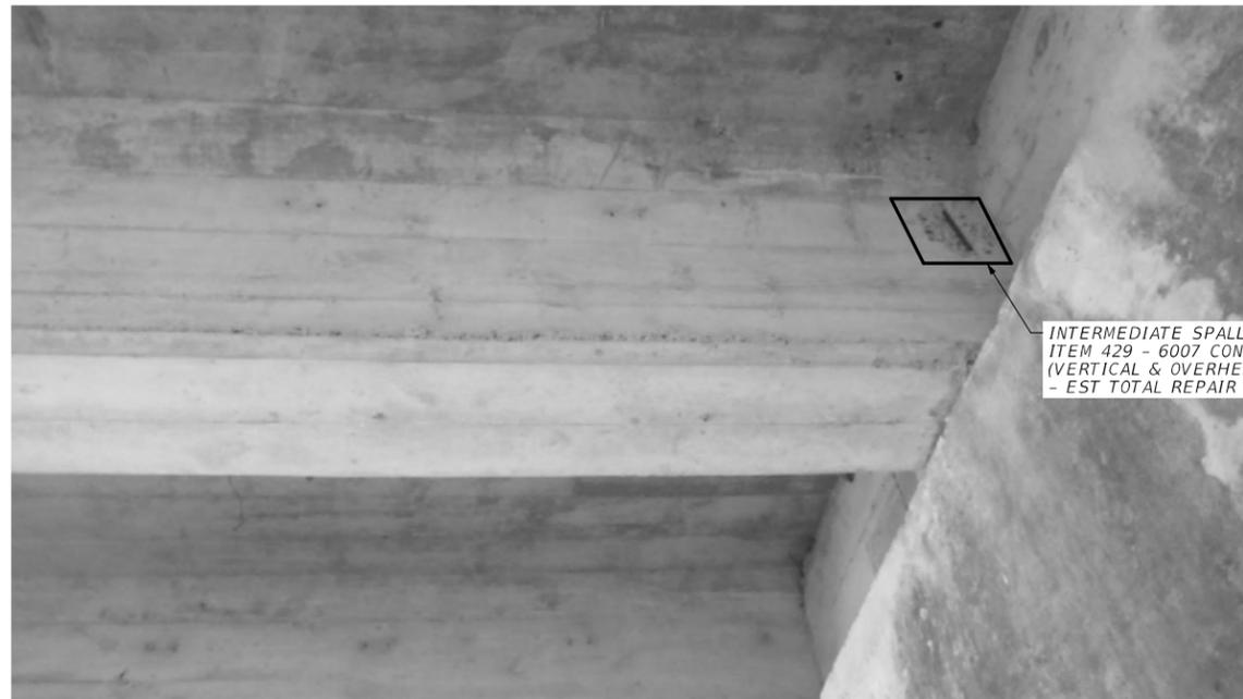
INTERMEDIATE SPALL REPAIR.
