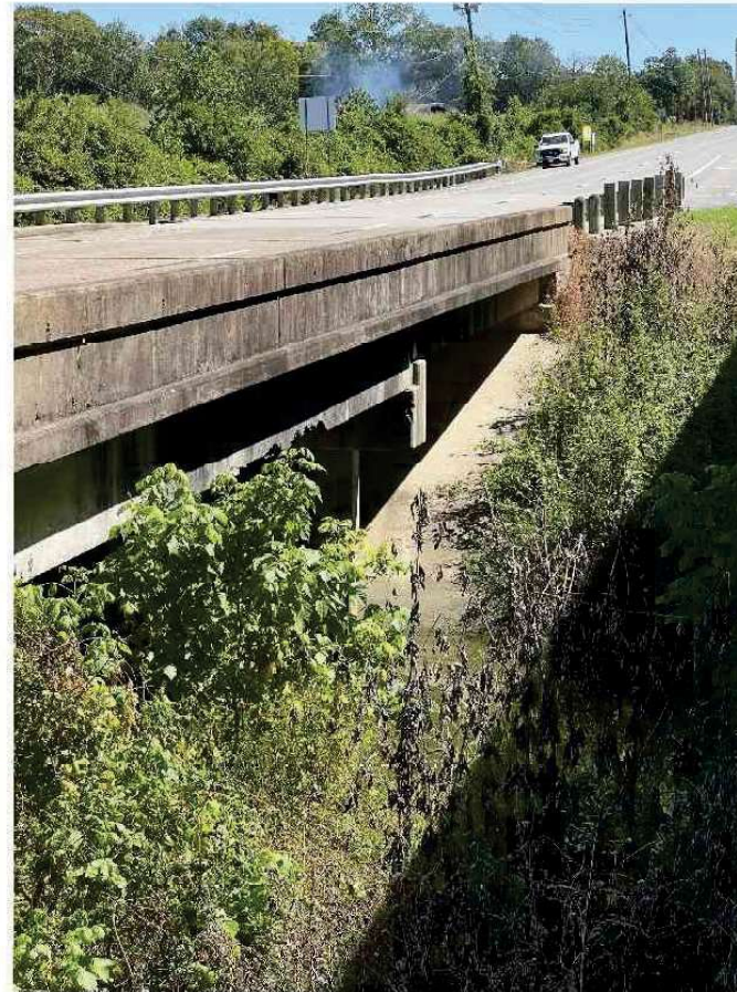
SPAN 2 - PAN GIRDER 1 (FROM SOUTH)
