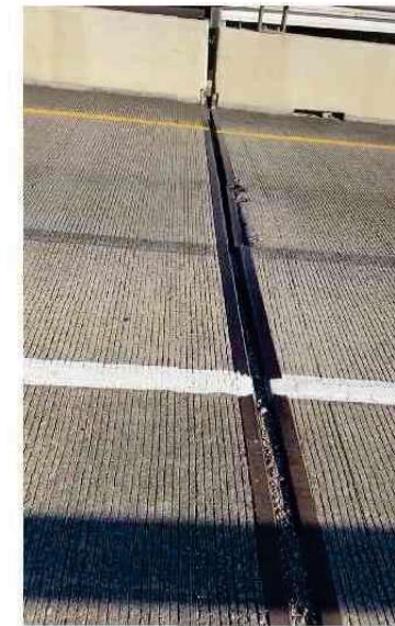
EXISTING JOINT AT BENT 29 PHOTO - 9/28/2022 WORK ZONE REPAIR #3
