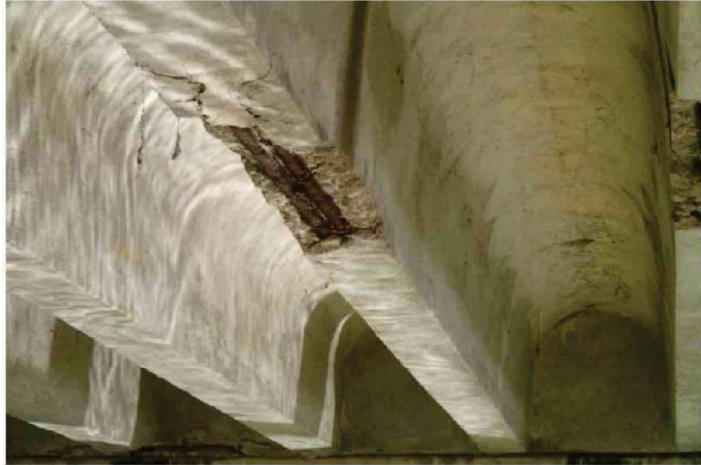
SPAN 1 - PAN GIRDER 3 (FROM SOUTH)
