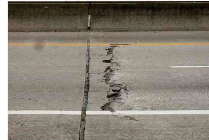
EXISTING NW APPROACH SLAB PHOTO - 10/13/2020
