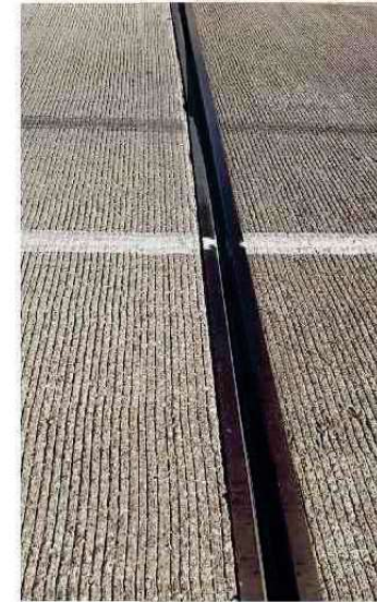
EXISTING JOINT AT BENT 24 PHOTO - 9/28/2022
