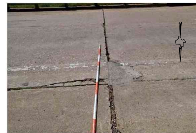
EAST APPROACH RELIEF JOINT PHOTO - 10/13/2020 WORK ZONE REPAIR #1
