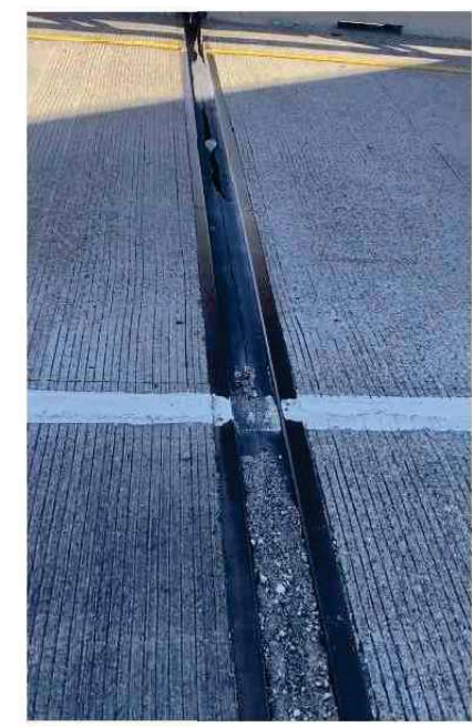
EXISTING JOINT AT BENT 21 PHOTO - 9/28/2022 WORK ZONE REPAIR #3
