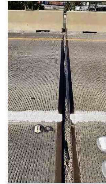
EXISTING JOINT AT BENT 6 PHOTO- 9/28/2022
