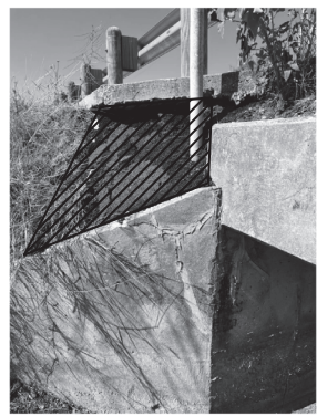
SOUTHEAST WINGWALL FLOWABLE BACKFILL 1 CY
