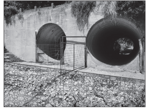
1 NORTHWEST RIPRAP 72 SY GABION MATTRESS
