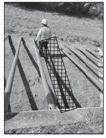
1 PIPE RUNNER 3 SOUTHWEST
