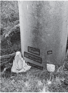
1 BENT 5 COLUMN 2 SQFT INTERMEDIATE SPALL REPAIR
