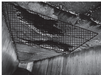
1 BOTTOM SLAB BARREL No. 9 64 SQFT INTERMEDIATE SPALL REPAIR
