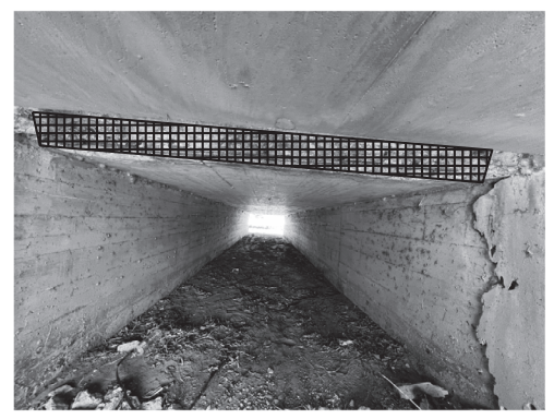
1 BARREL No. 5 14 SQFT INTERMEDIATE SPALL REPAIR
