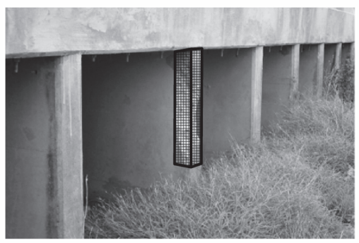
① INTERIOR WALL No. 8 4.5 SQFT INTERMEDIATE SPALL REPAIR
