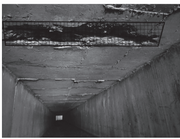
3 BOTTOM TOP SLAB BARREL No. 3 12 SQFT INTERMEDIATE SPALL REPAIR
