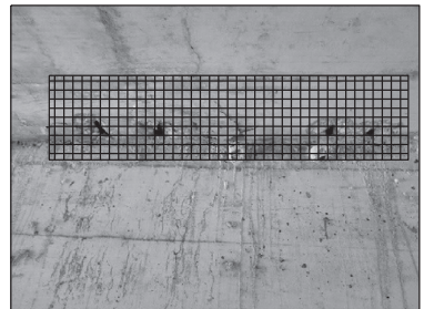
1 BOTTOM TOP SLAB BARREL No. 6 5 SQFT INTERMEDIATE SPALL REPAIR
