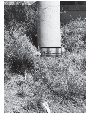
2 BENT 5 COLUMN 4 SQFT INTERMEDIATE SPALL REPAIR
