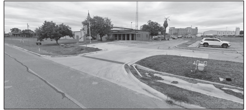
SITE 2 - COTULLA MAINTENANCE OFFICE
