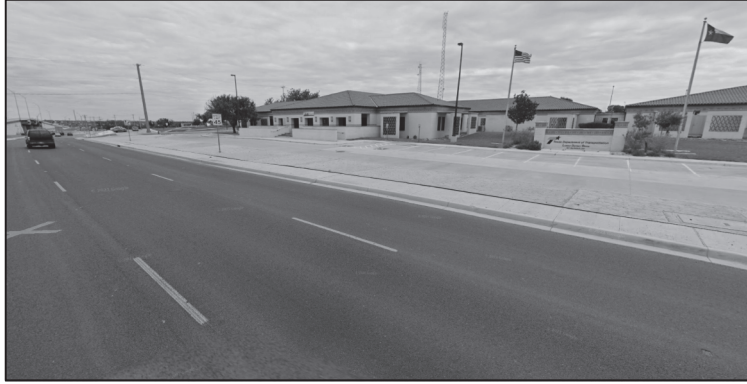
SITE 1 - LAREDO MAINTENANCE OFFICE
