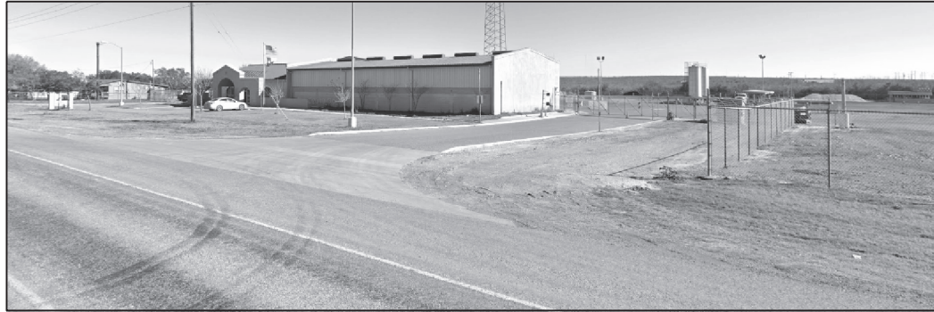
SITE 3 - FREER MAINTENANCE OFFICE
