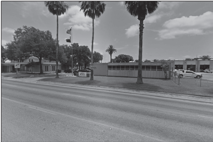
SITE 3 - DEL RIO MAINTENANCE OFFICE
