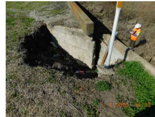
Pic. 7 Wingwall Repair (NW Wingwall)
