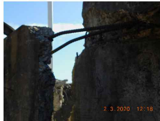
Pic. 6 Wingwall Repair (NW Wingwall)
