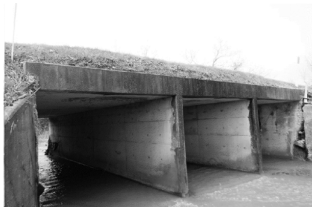
PIC:1 - LOOKING NORTH UPSTREAM VIEW
