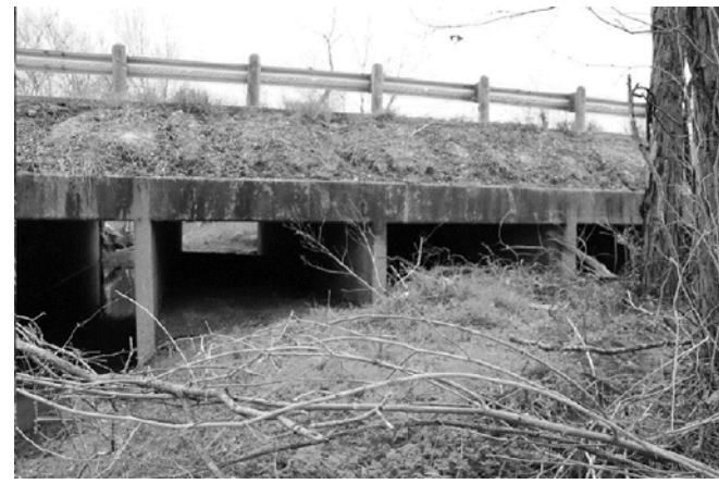
PIC:2 - LOOKING NORTHEAST STREAM UNDER BRIDGE DEBRIS CLEAN - UPSTREAM
