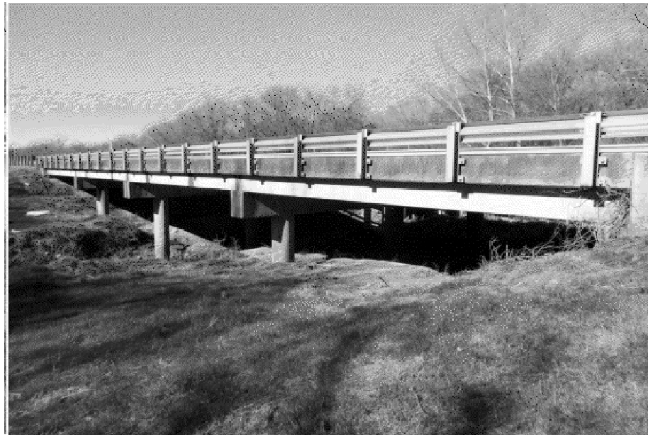
PIC:1 - BRIDGE ELEVATION LOOKING NORTHWEST
