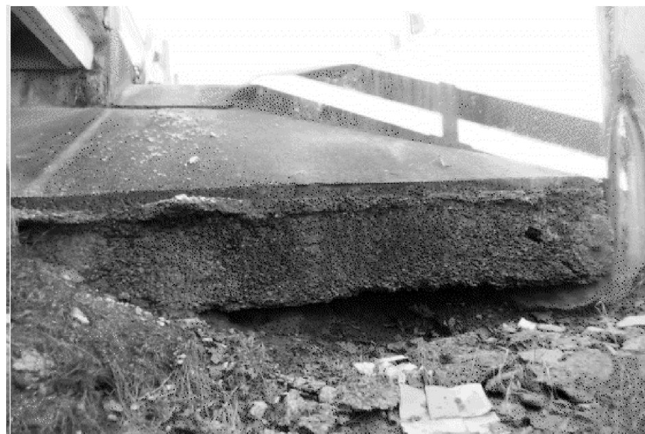
PIC:4 - LOOKING WEST NW CORNER RIPRAP BACKFILL 4' OF UNDERMINING FLOWABLE BACKFILL (8' +)
