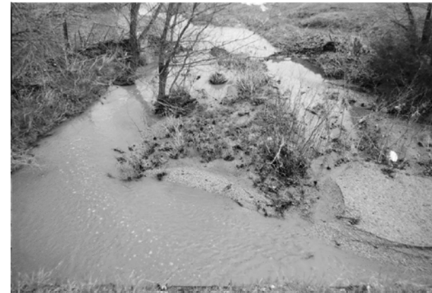
PIC:3 - LOOKING SOUTHEAST DOWNSTREAM FROM BRIDGE DEBRIS CLEAN & CHANNEL RESHAPE
