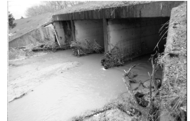
PIC:4 - LOOKING EAST UPSTREAM NORTH WINGWALL REPAIR & DEBRIS CLEAN
