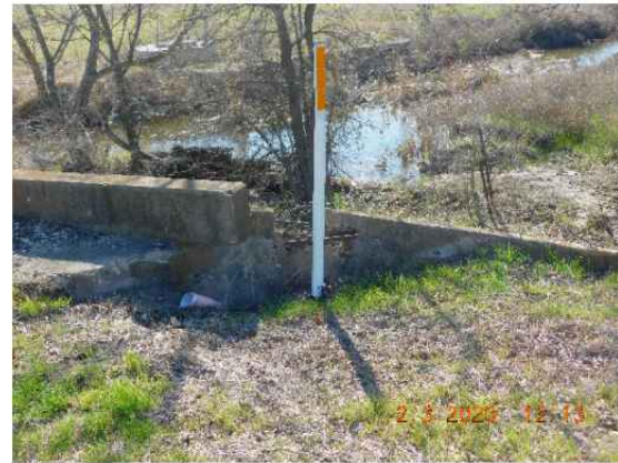
Pic. 2 Wingwall Repair (SE Wingwall)
