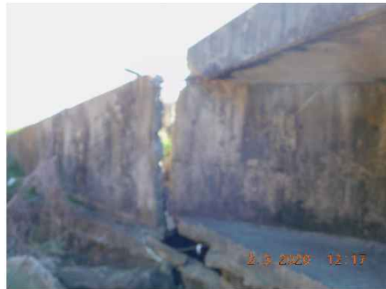
Pic. 5 Wingwall Repair (NW Wingwall)
