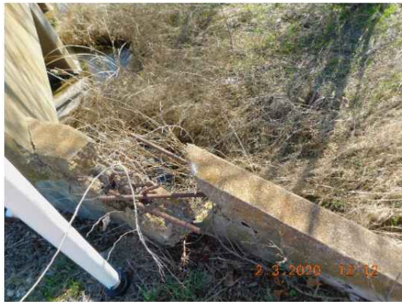
Pic. 1 Wingwall Repair (SE Wingwall)
