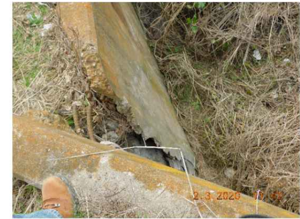
Pic. 4 Wingwall Repair (SE Wingwall)
