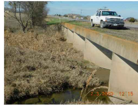
Pic. 3 Box Clean Up & Reshaping The Channel (Up Stream)
