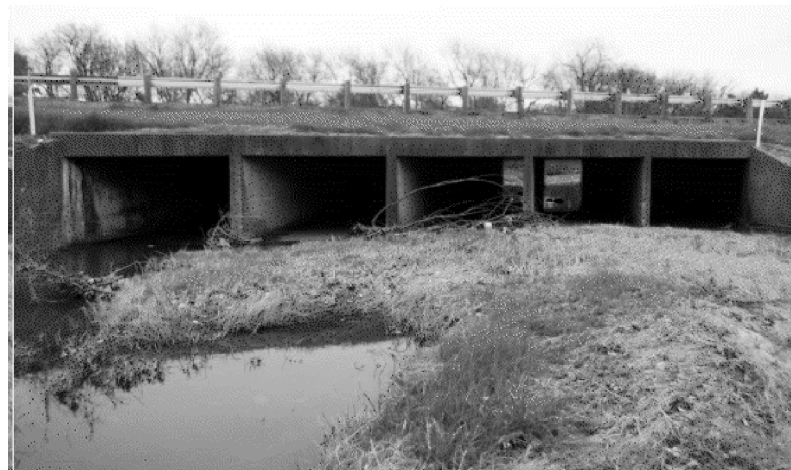
PIC:3 - LOOKING NORTH UPSTREAM DITCH RESHAPE DITCH
