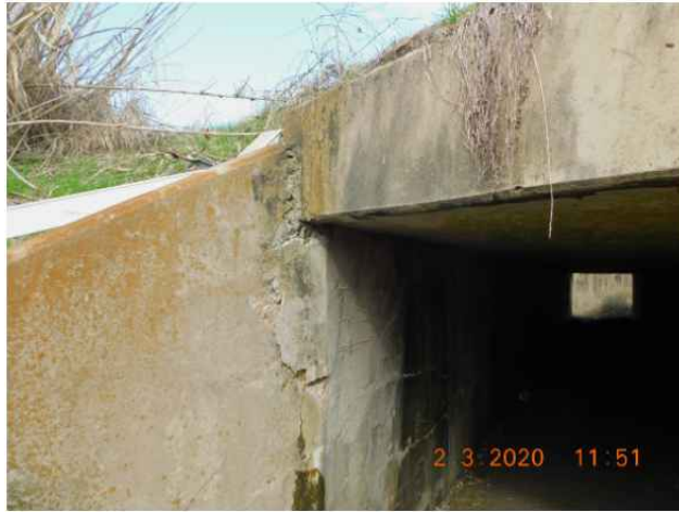
Pic. 1 Concrete Repair At SW Wingwall (Vertical & Overhead)
