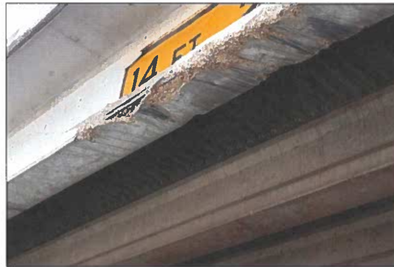
⑤ EXPOSED STRAND BEAM 1 FROM NORTH SPAN 4
