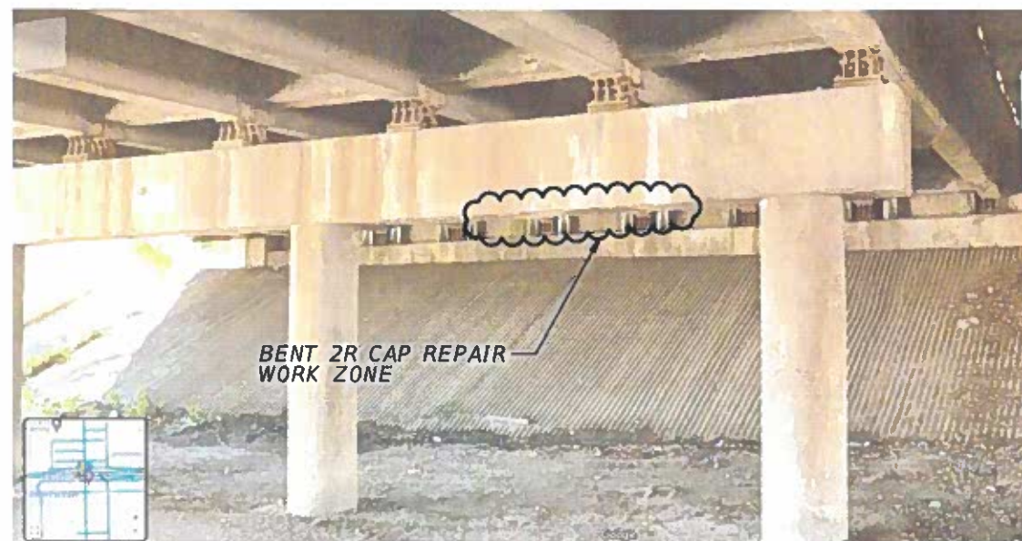
BENT 2R BENT OVERVIEW PHOTO GOOGLE STREET VIEW ~ LOOKING WEST
