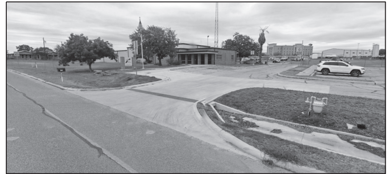
SITE 2 - COTULLA MAINTENANCE OFFICE
