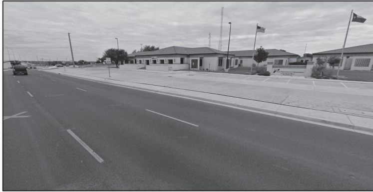
SITE 1 - LAREDO MAINTENANCE OFFICE
