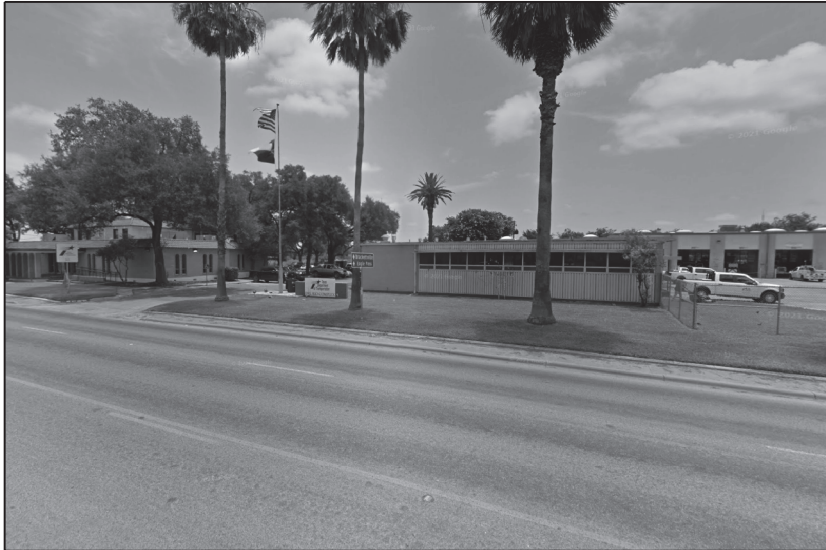
SITE 3 - DEL RIO MAINTENANCE OFFICE
