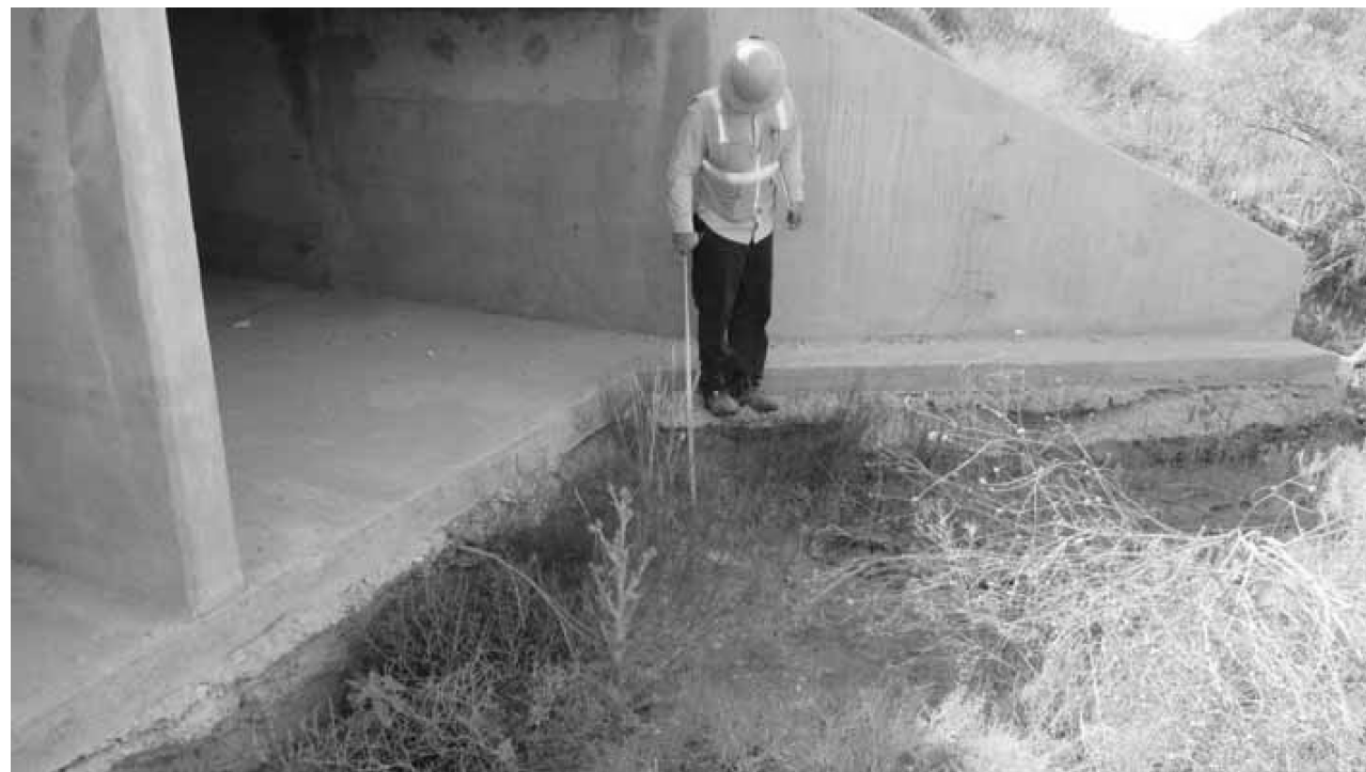
UPSTREAM CHANNEL BED - LOOKING SOUTHEAST
