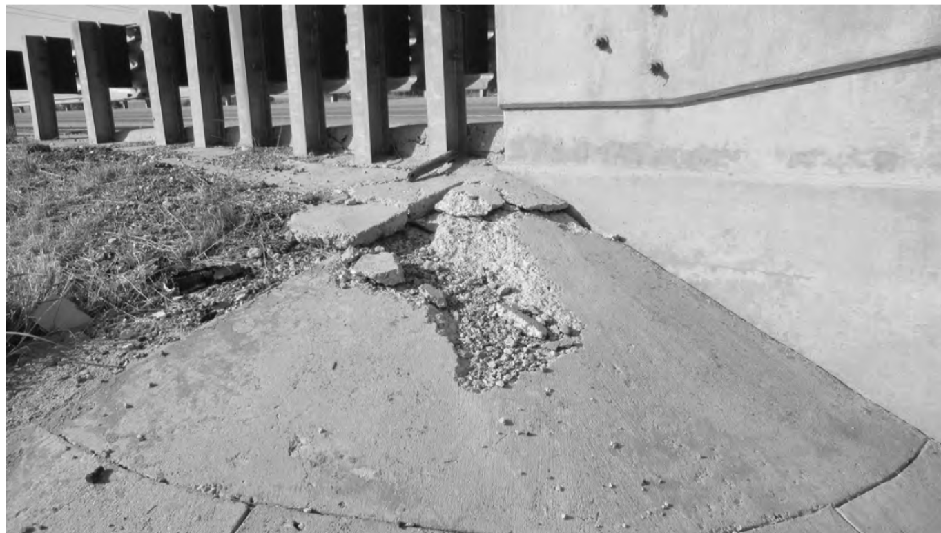
EAST EMBANKMENT - LOOKING SOUTHEAST
