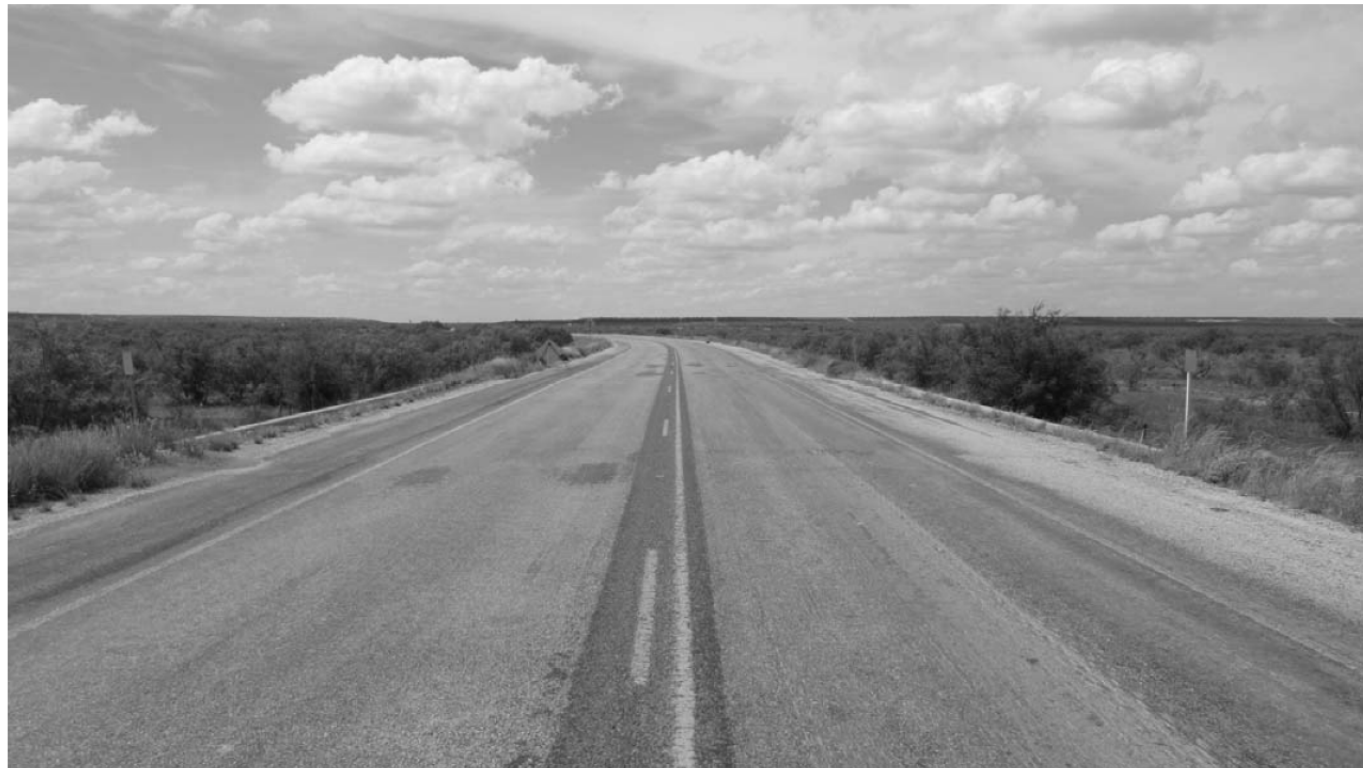
ROADWAY VIEW - LOOKING SOUTH
