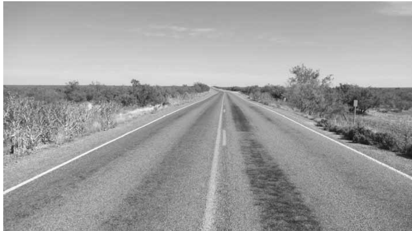
ROADWAY VIEW - LOOKING NORTHWEST
