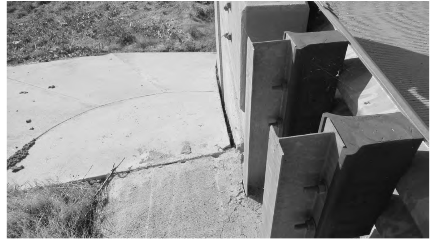
NORTH EMBANKMENT - LOOKING SOUTHEAST
