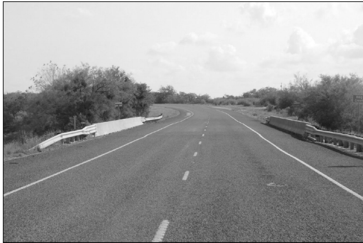
ROADWAY VIEW US 67 Looking NE IMG 1947
