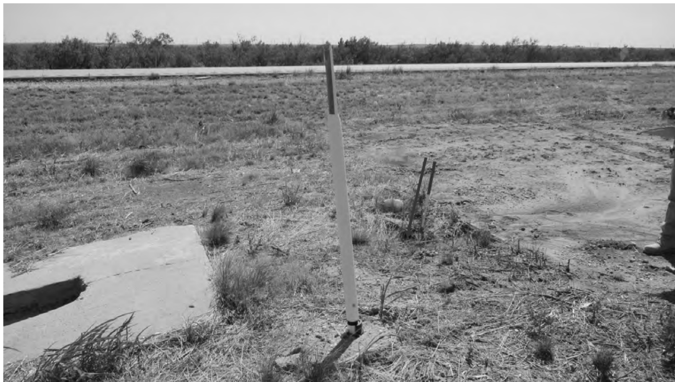
MEDIAN DITCH - LOOKING WEST
