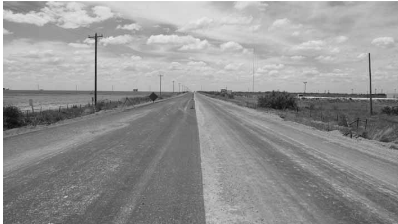
ROADWAY VIEW - LOOKING SOUTH
