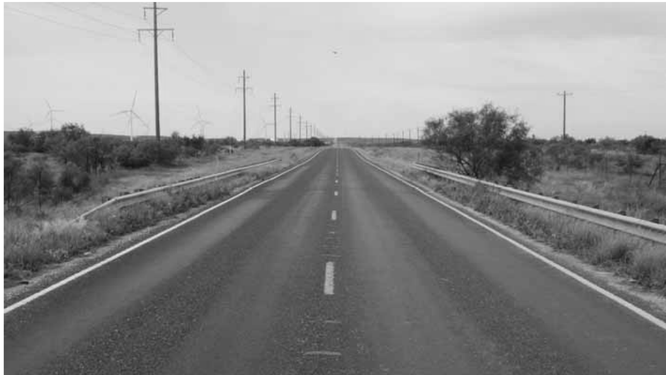
ROADWAY VIEW - LOOKING SOUTH
