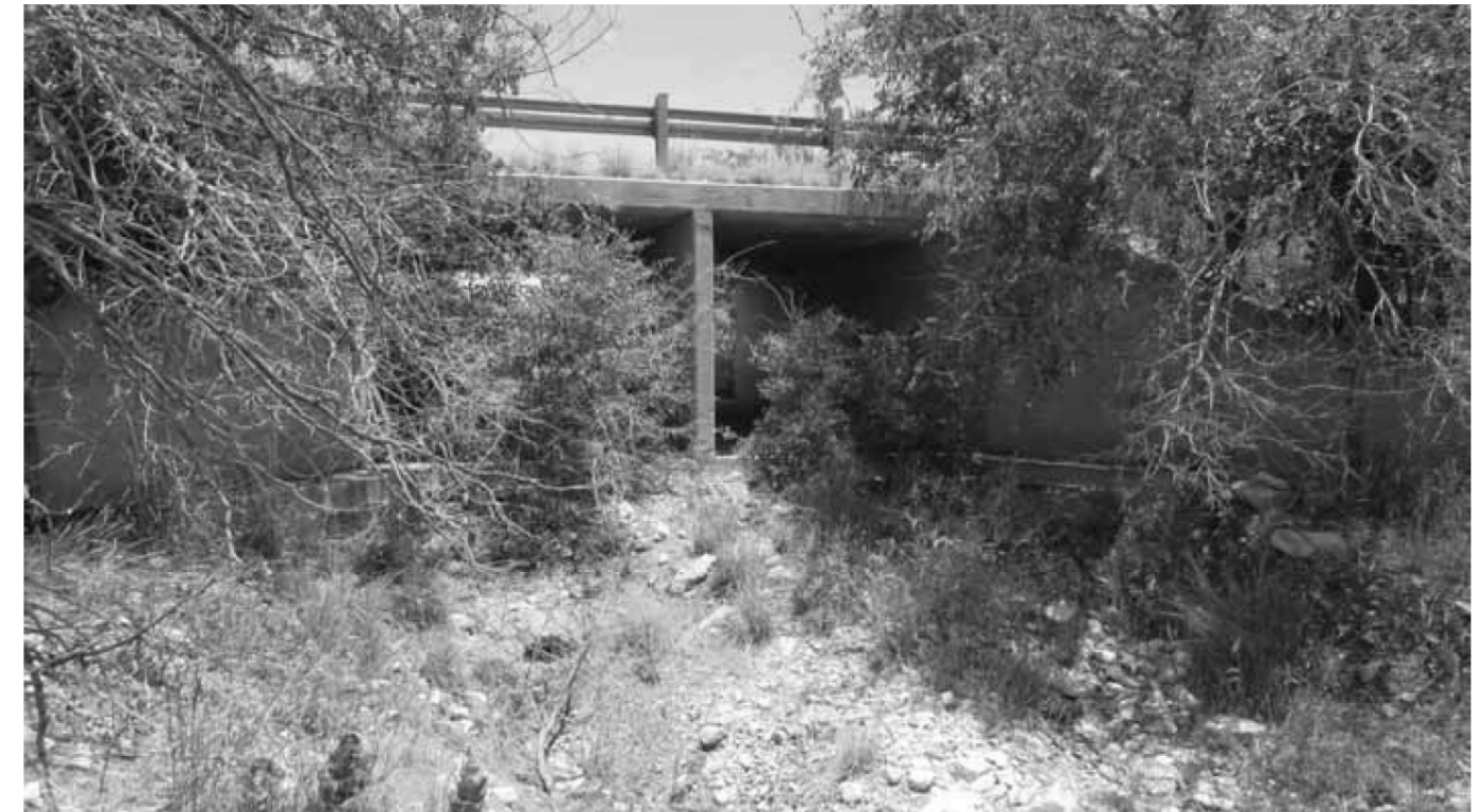
ELEVATION VIEW - LOOKING SOUTHEAST
