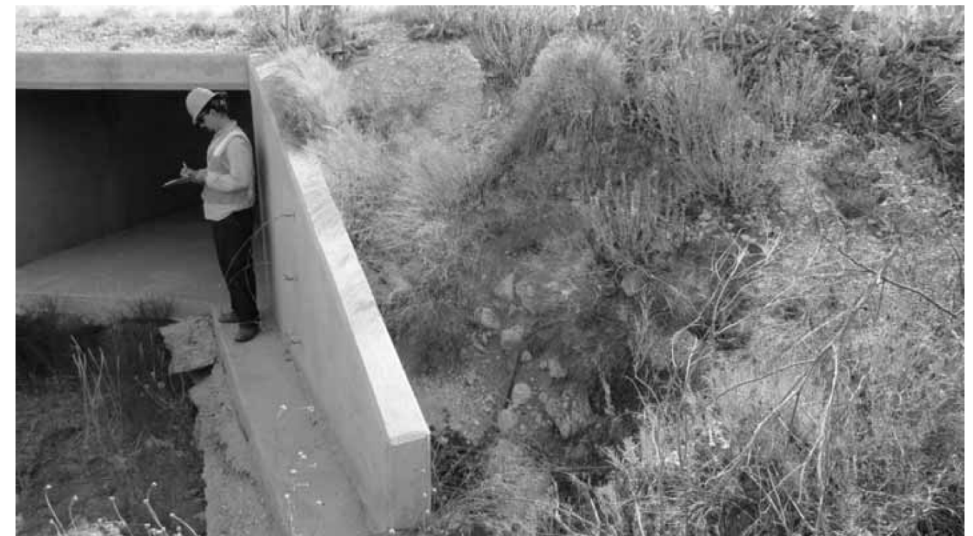
SOUTH EMBANKMENT - LOOKING NORTHEAST
