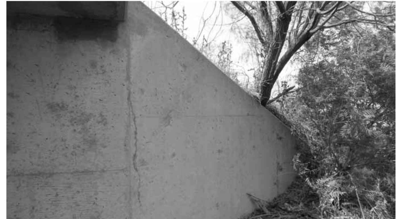
SOUTHWEST WINGWALL - LOOKING SW
