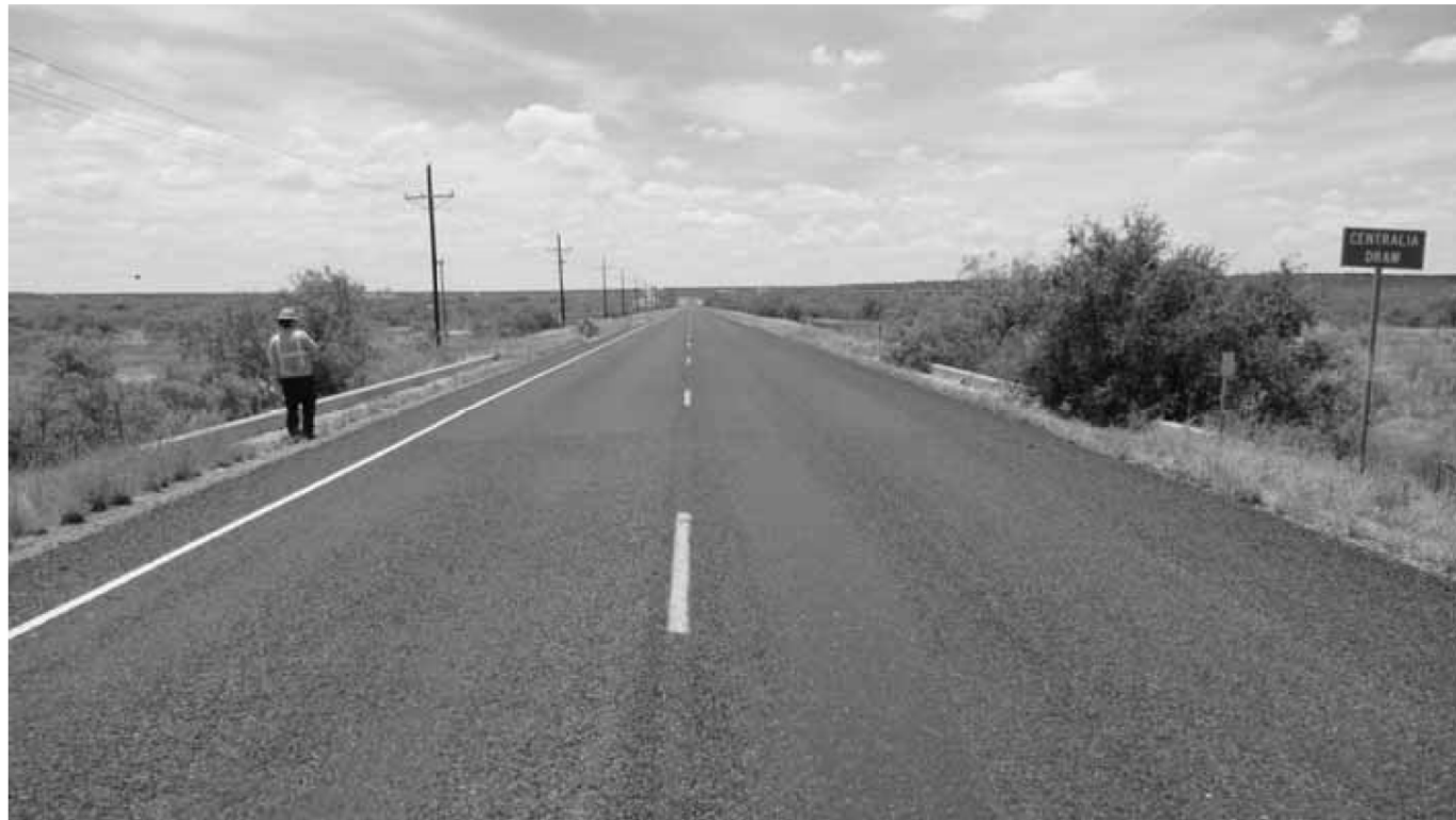
ROADWAY VIEW - LOOKING SOUTH
