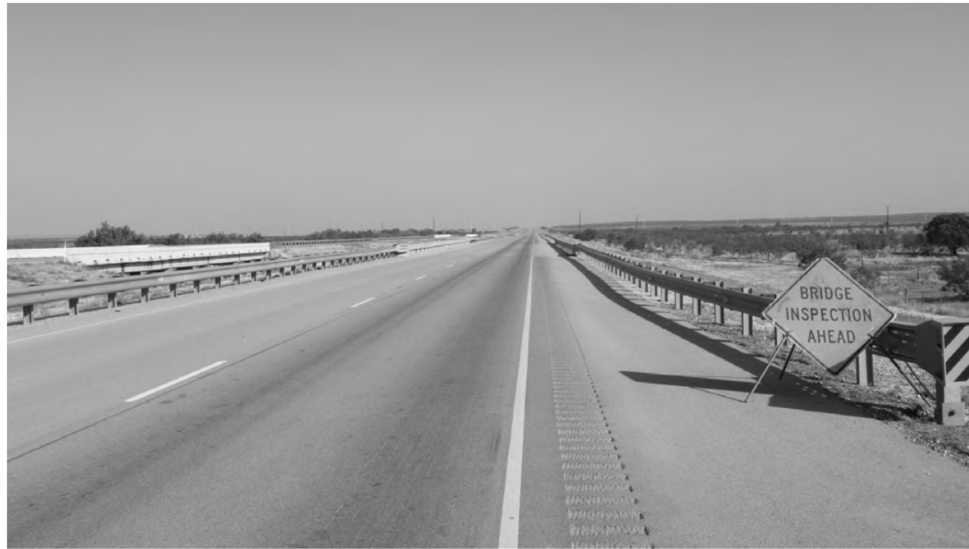
ROADWAY VIEW - LOOKING NORTHWEST
