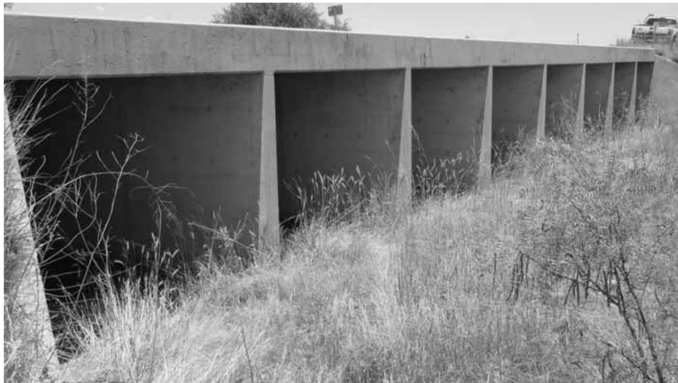
ELEVATION VIEW - LOOKING NORTHWEST
