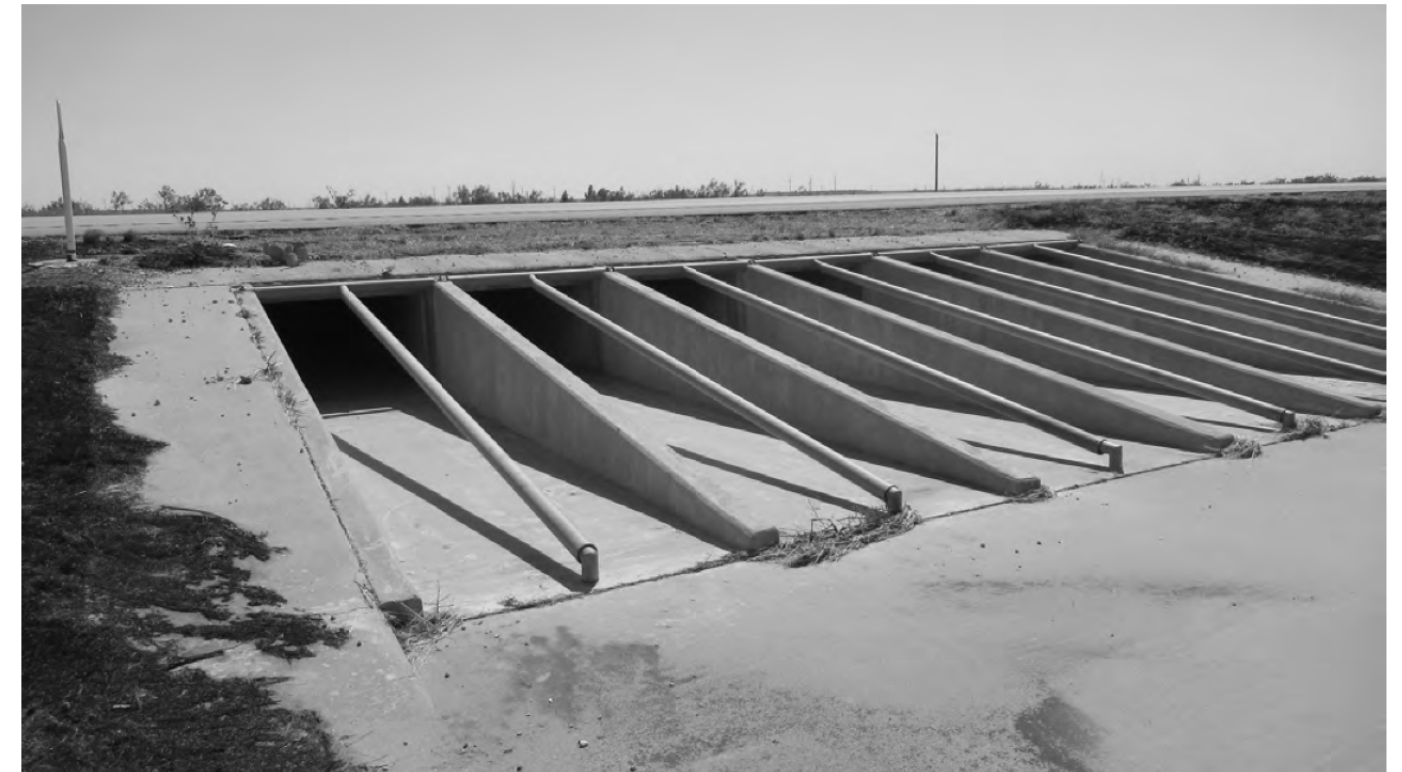
ELEVATION VIEW - LOOKING WEST
