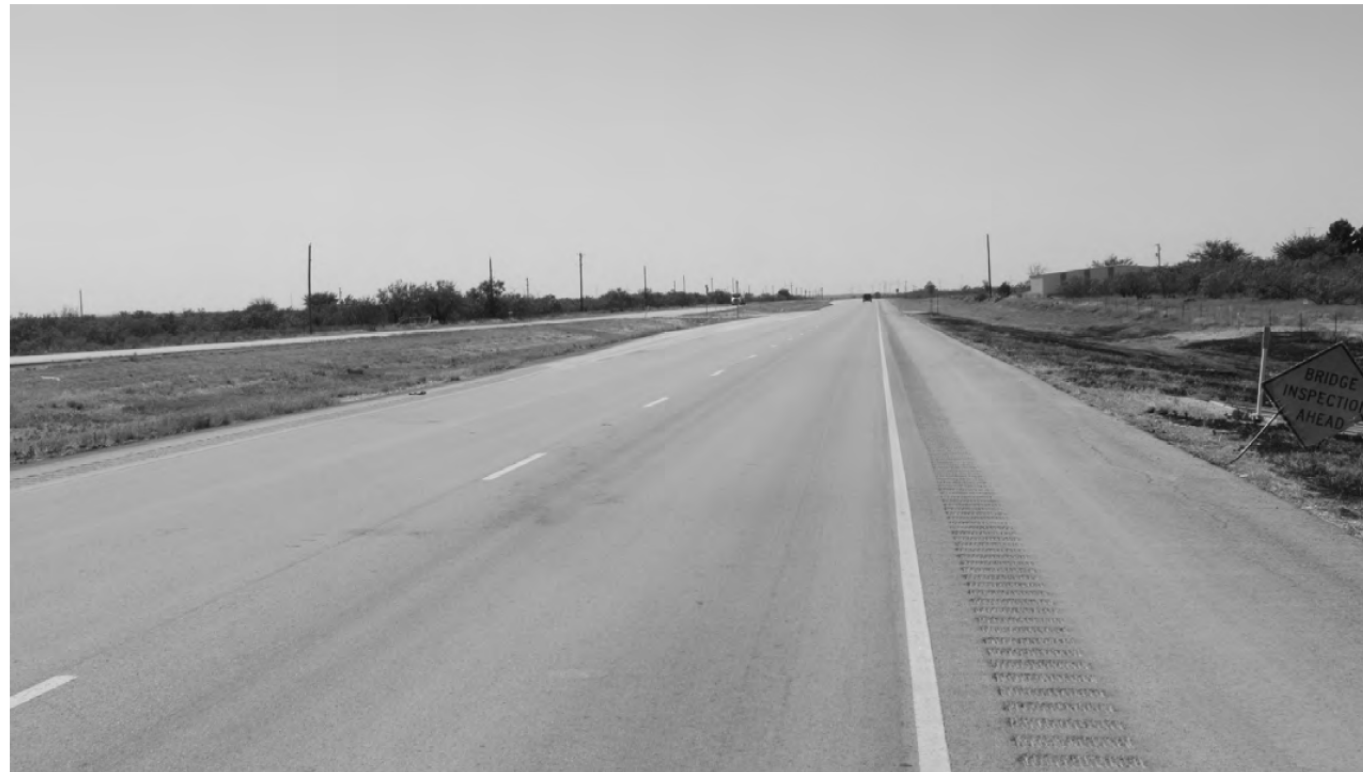
ROADWAY VIEW - LOOKING NORTHWEST
