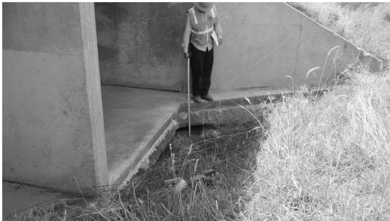
UPSTREAM CHANNEL BED - LOOKING SOUTH
