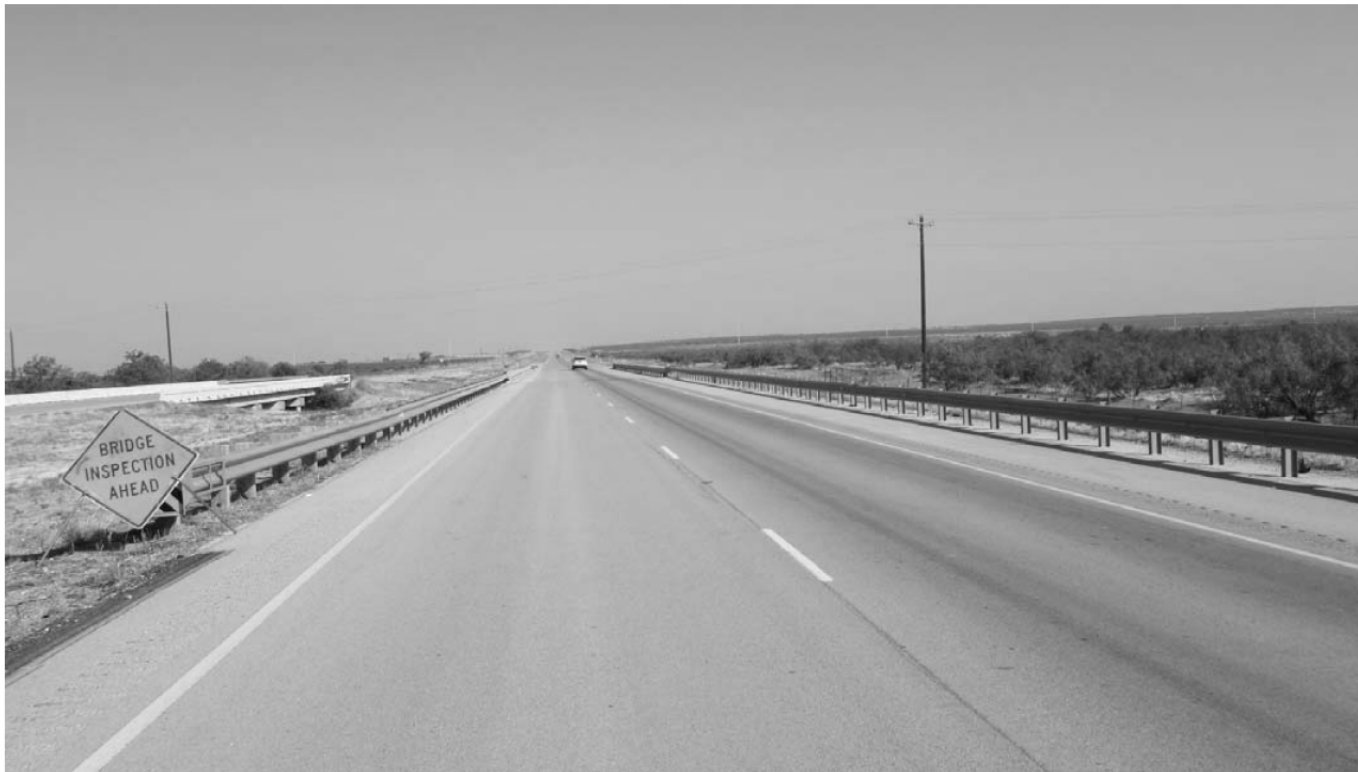
ROADWAY VIEW - LOOKING NORTHWEST VIEW 3941
