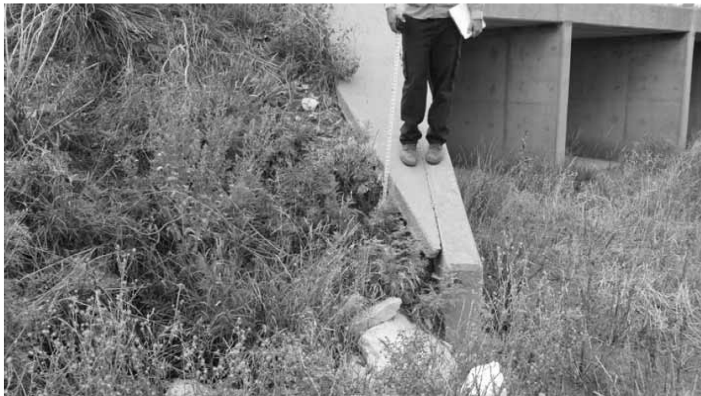
NORTHWEST EMBANKMENT - LOOKING SOUTHEAST
