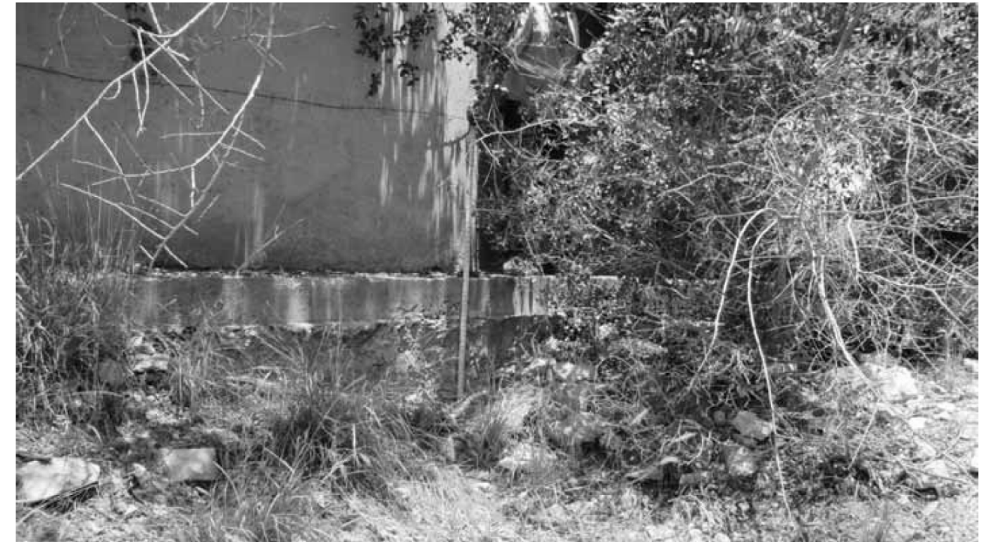
NORTHWEST WINGWALL - LOOKING NORTHEAST
