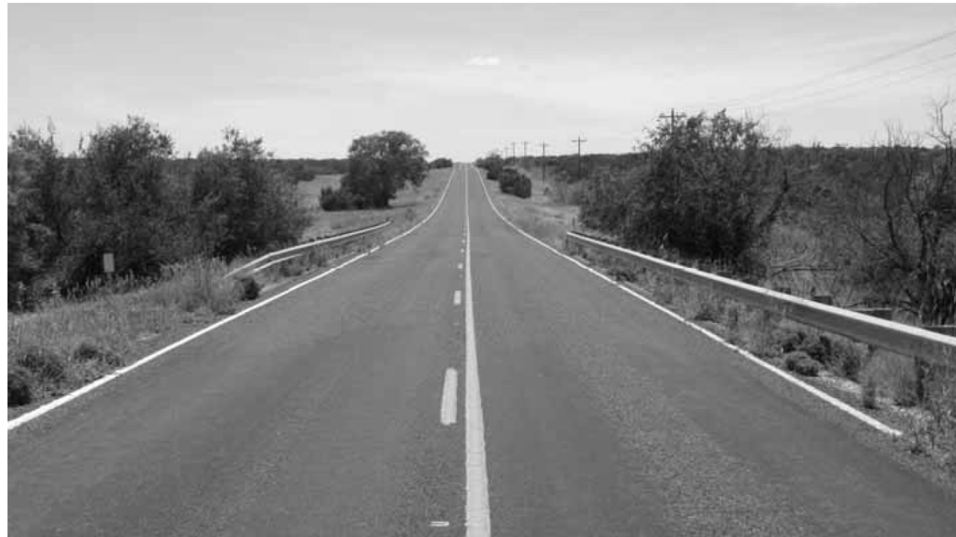
ROADWAY VIEW - LOOKING SOUTH
