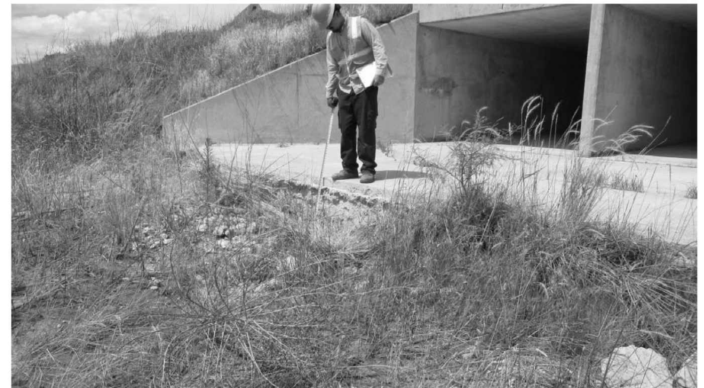
DOWNSTREAM APRON - LOOKING SOUTHWEST
