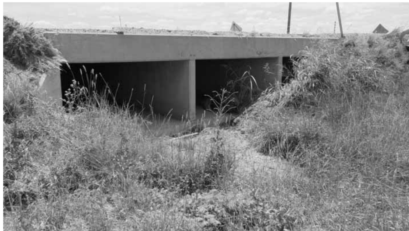
ELEVATION VIEW - LOOKING SOUTHEAST
