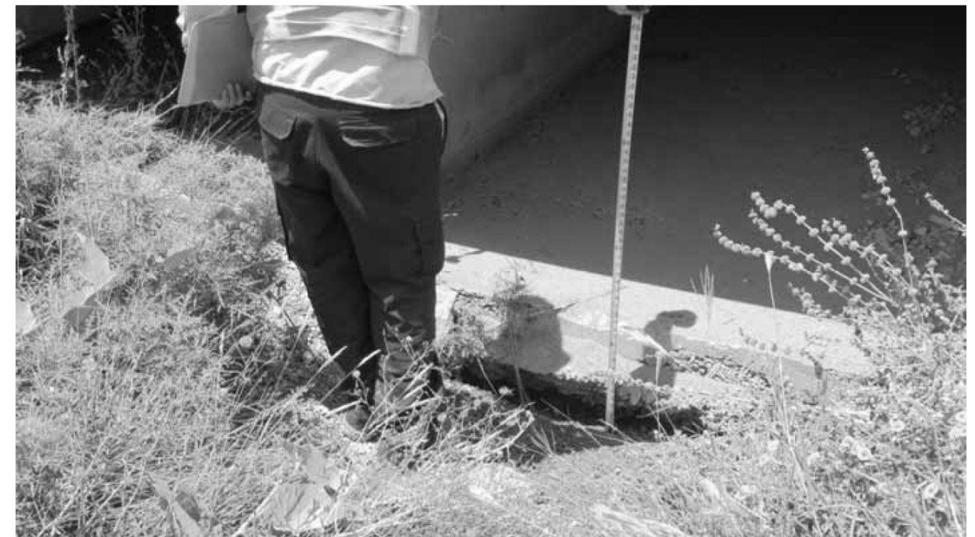
UPSTREAM CHANNEL BED - LOOKING WEST
