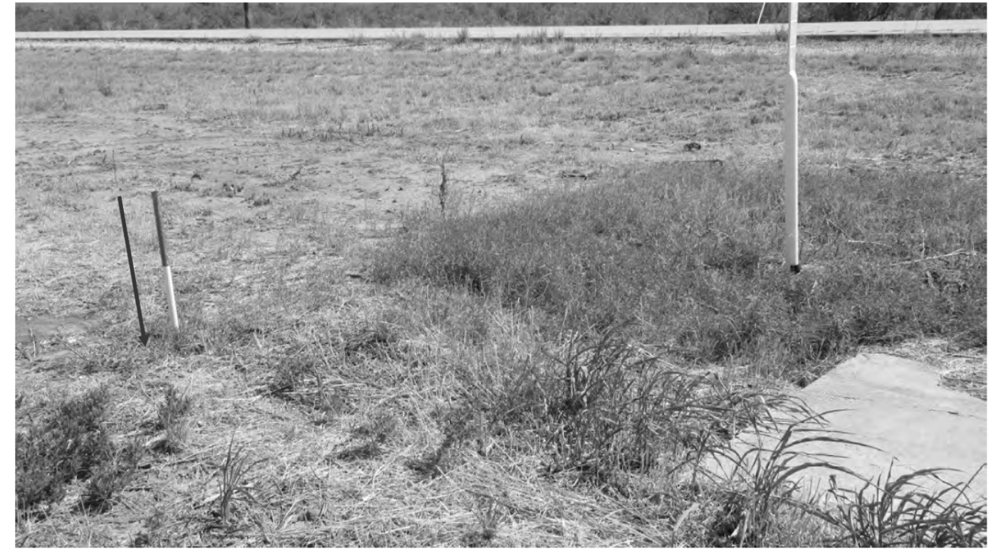
MEDIAN DITCH - LOOKING SOUTH
